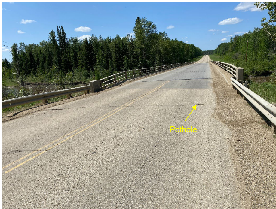
Photo 12: Pavement surface at east abutment. Looking west.
