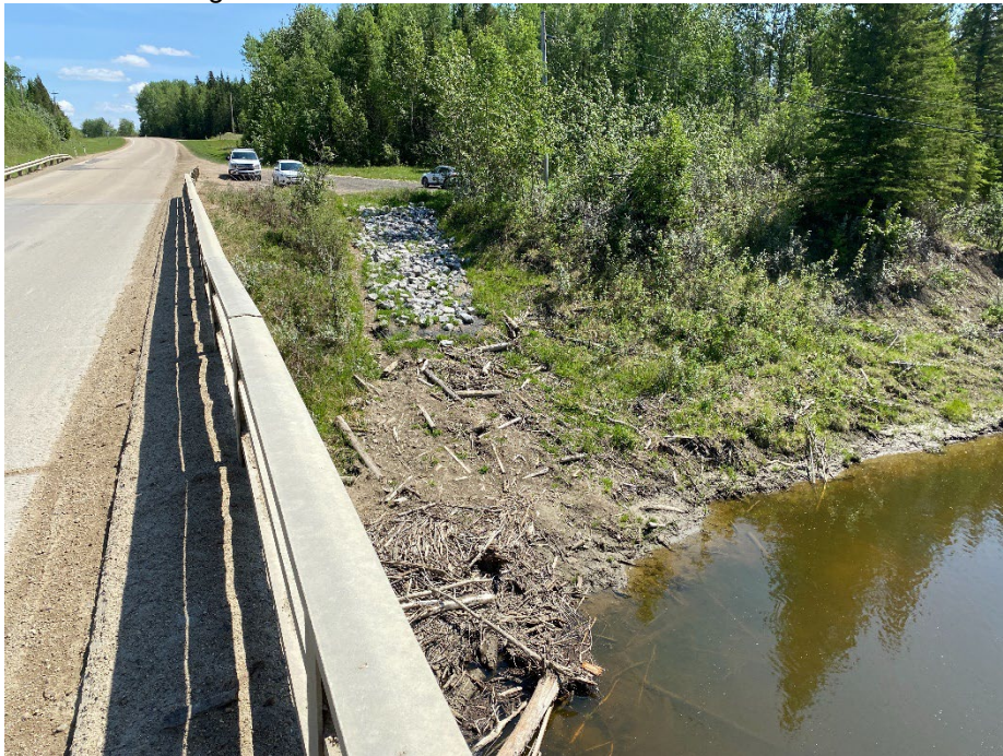
Photo 10: Riprap placed south of bridge along previous erosion channel. Looking southeast.
