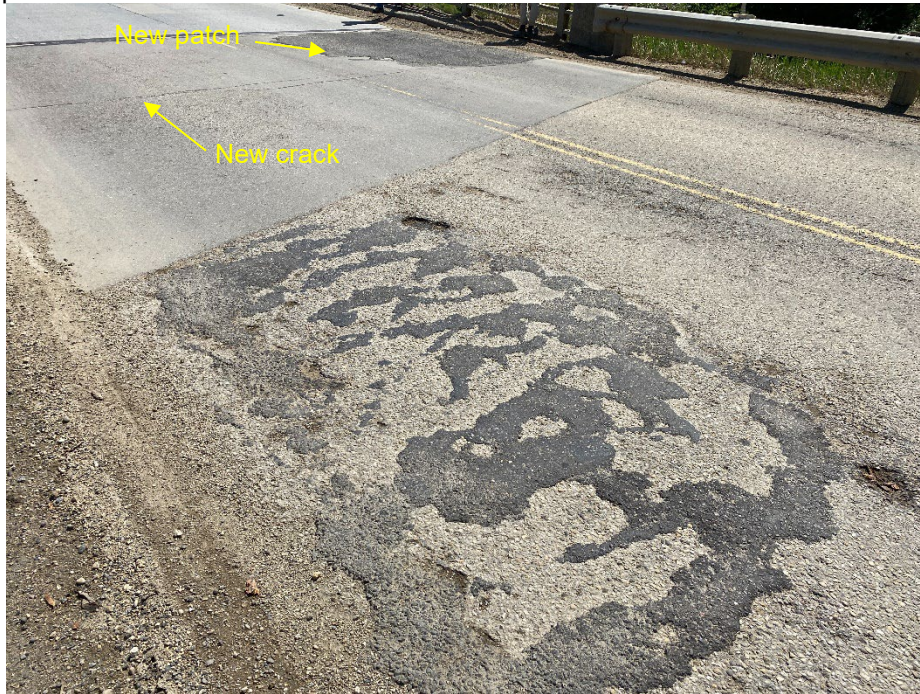
Photo 11: Pavement surface at west abutment. Looking southeast.
