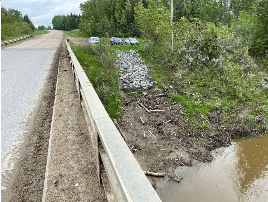
Photo 9: Riprap placed south of bridge along previous erosion channel. Looking southeast.
