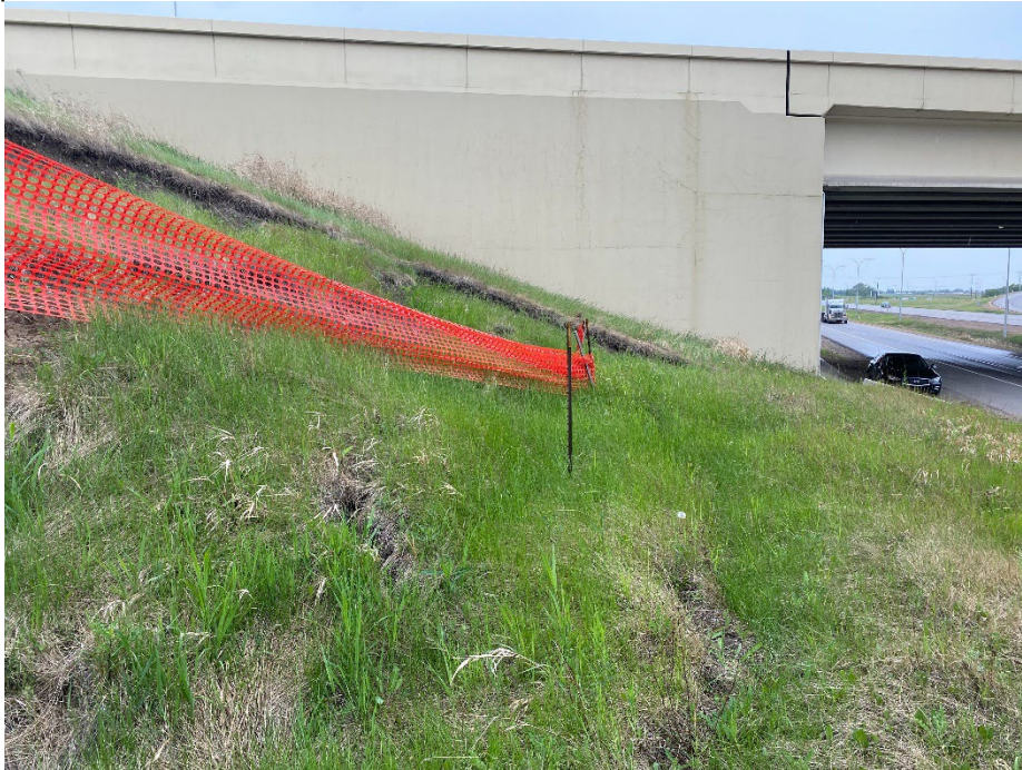
Photo 3: Mid slope of slump on south embankment. Looking west.
