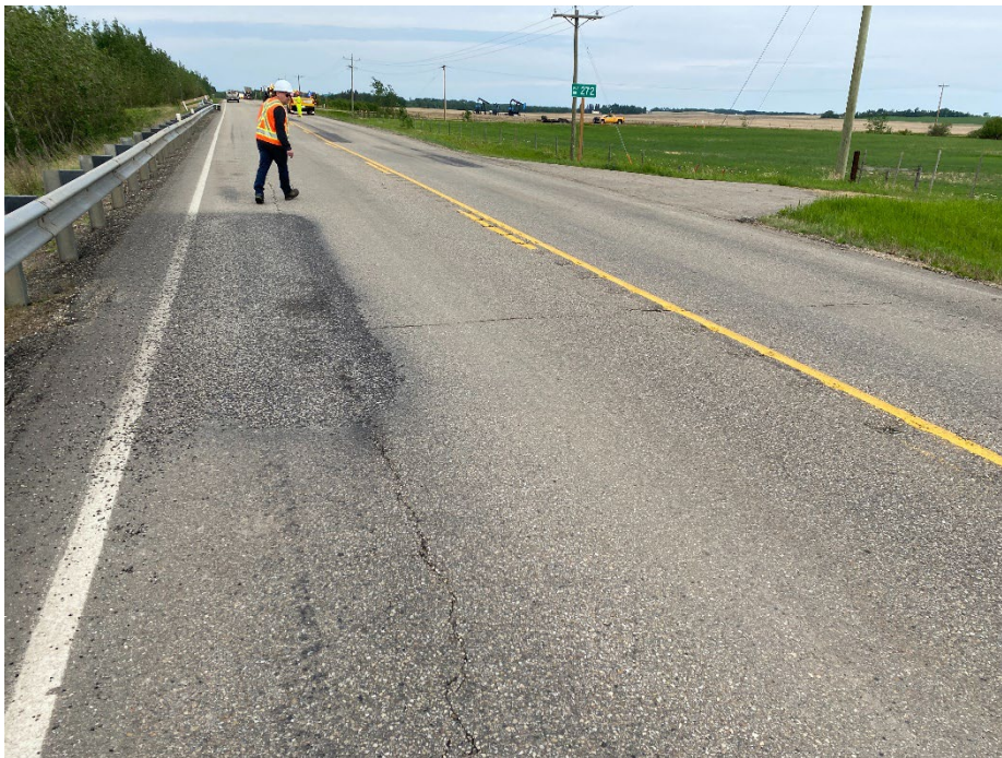
Photo 6: Highway surface above culvert. Looking west.
