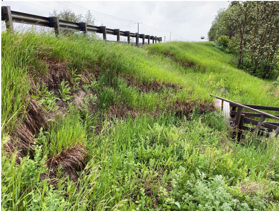
Photo 3: Scarp at west slump. Looking east.
