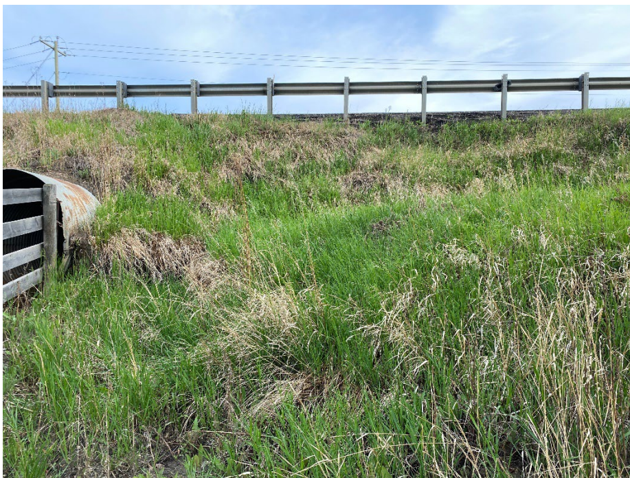
Photo 4: Possible regraded area on east side of culvert. Looking north.
