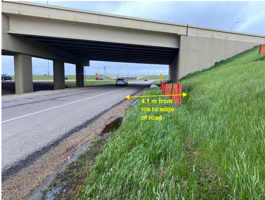
Photo 5: Toe of the embankment. Looking east.
