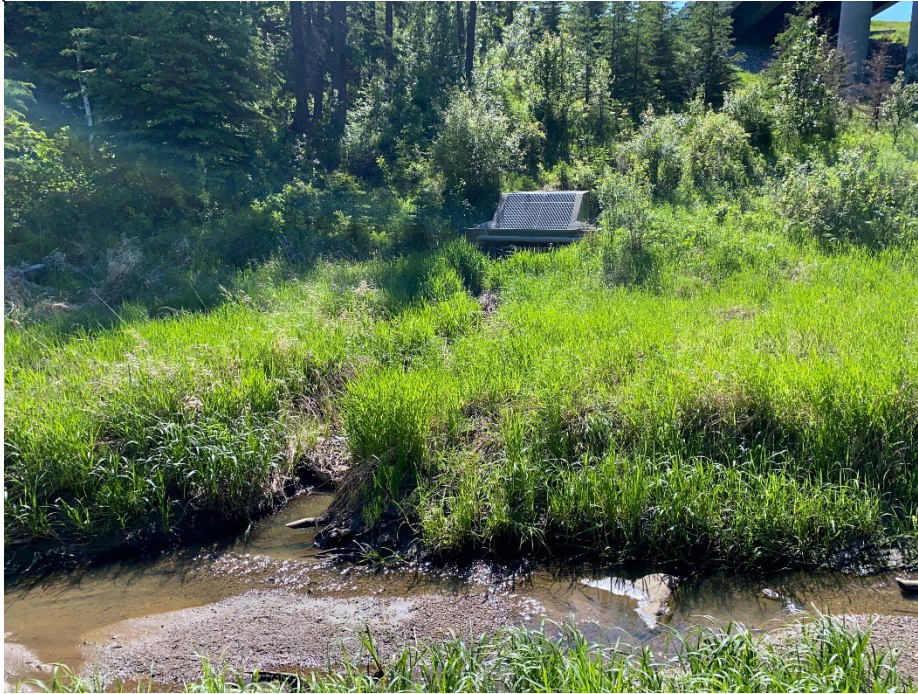
Photo 9: East outfall. Looking southeast.
