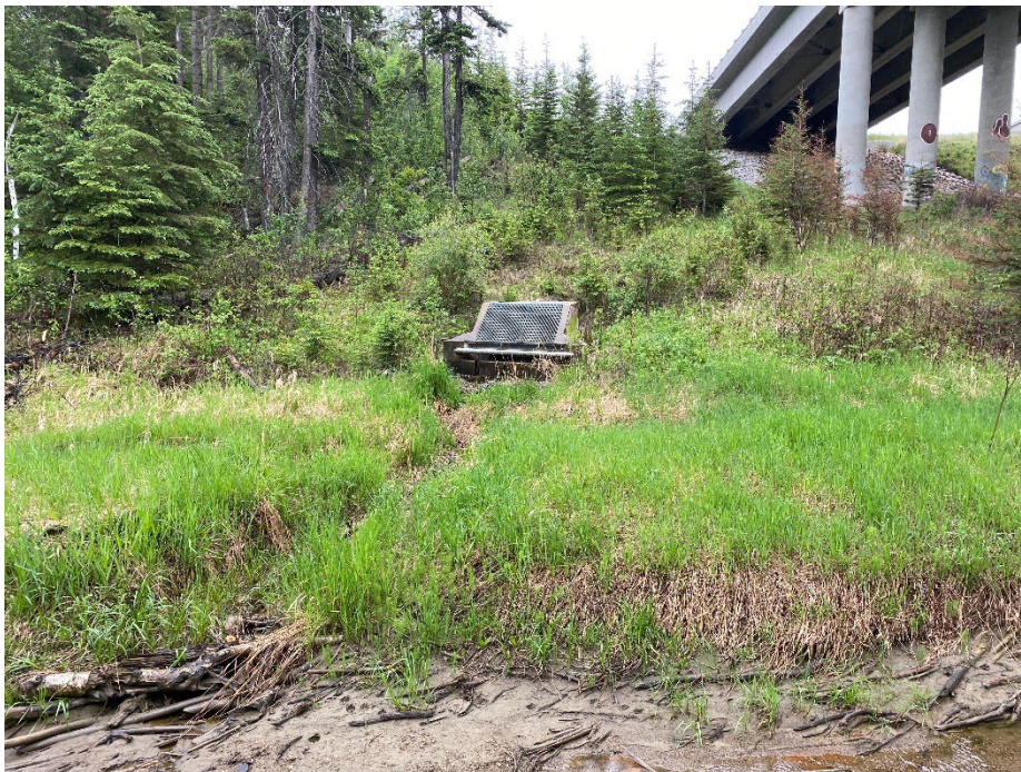
Photo 8: East outfall. Looking southeast.
