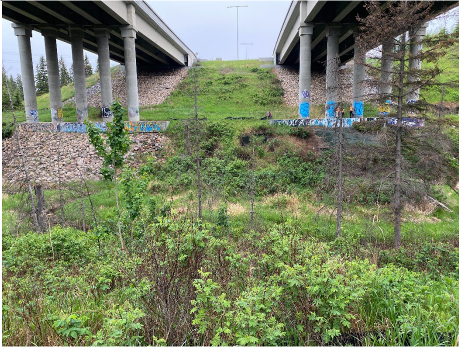
Photo 9: West slope with two slumps between pedestals and erosion mat exposed below northernmost pedestal. Looking northwest.
