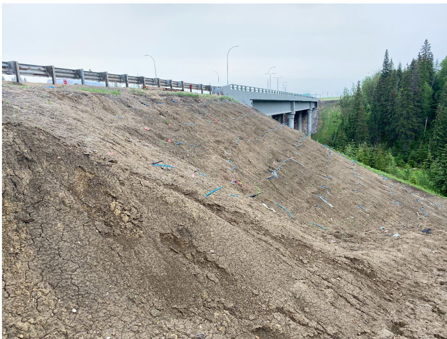
Photo 2: Soil nailed slope at north and south slide area. Looking southeast.
