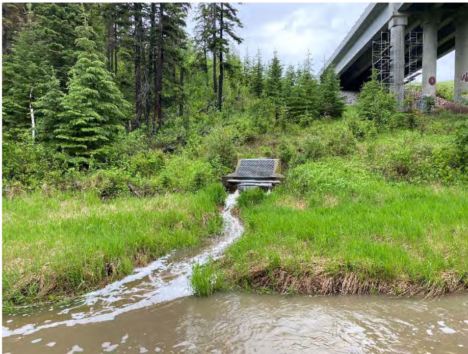
Photo 8: East outfall. Looking southeast.
