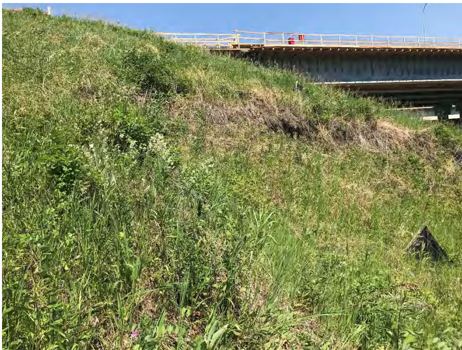
Photo 4: Scarp at south slide. Looking northeast.
