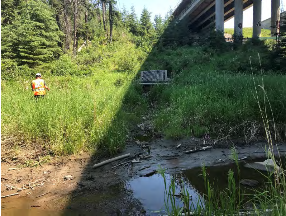
Photo 11: East outfall. Looking southeast.
