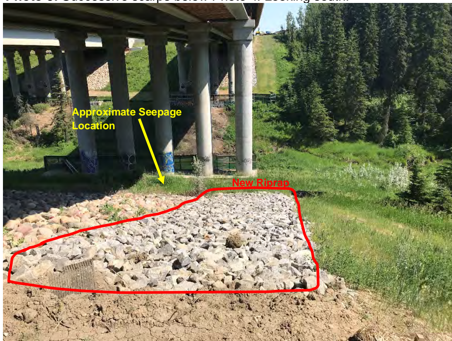
Photo 6: Riprap extended under southbound lane. Looking southeast.
