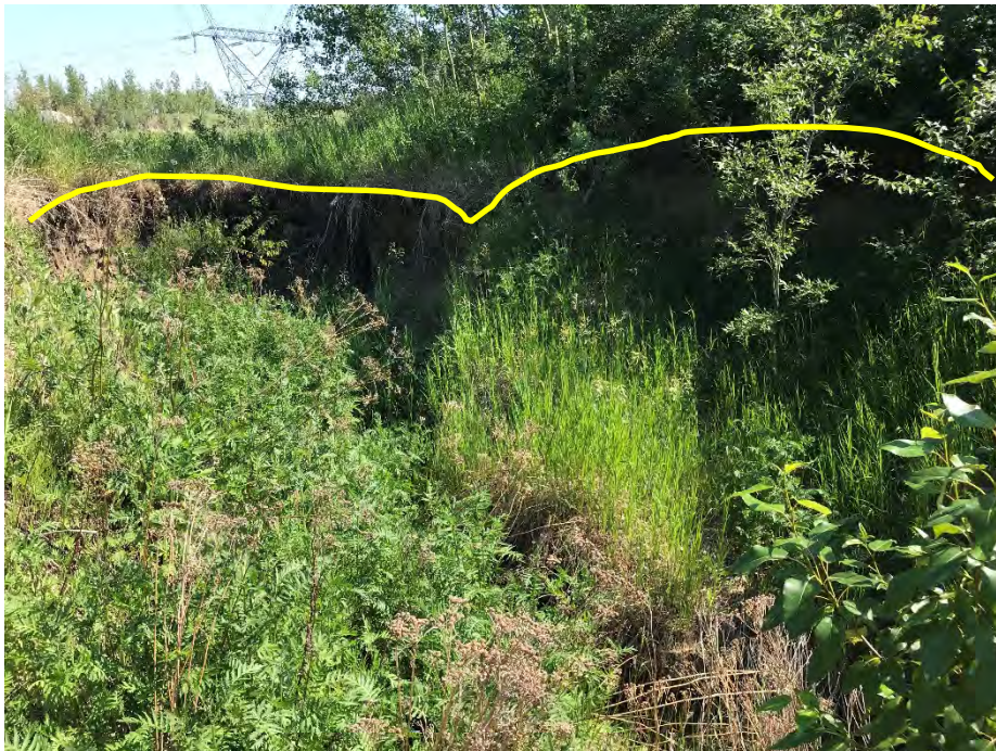
Photo 6: Two bowl shaped slumps adjacent and behind the outfall on the south bank of the river. Looking southeast.
