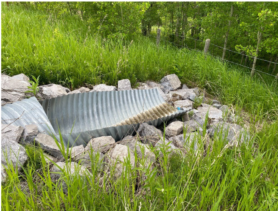
Photo 6: Culvert outlet south of the pile wall. Looking northeast.
