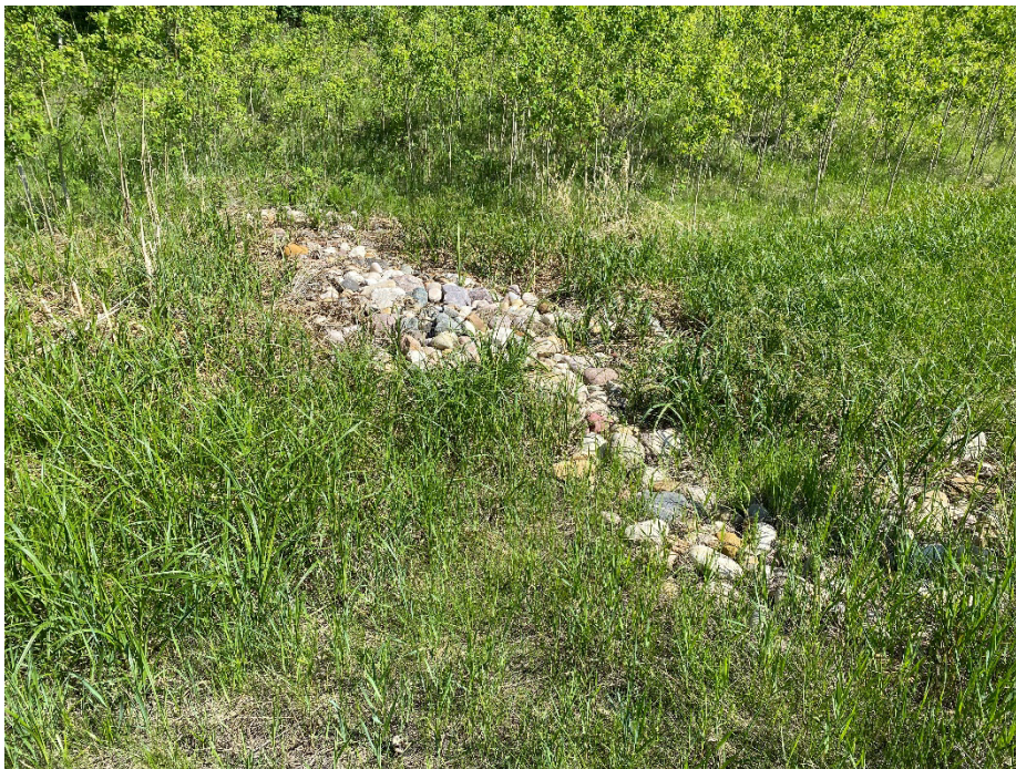
Photo 6: West most rock check dam in north ditch partially obscured by vegetation. Looking northeast.
