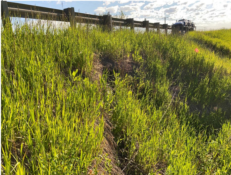
Photo 3: Scarp at west slump. Looking northeast.
