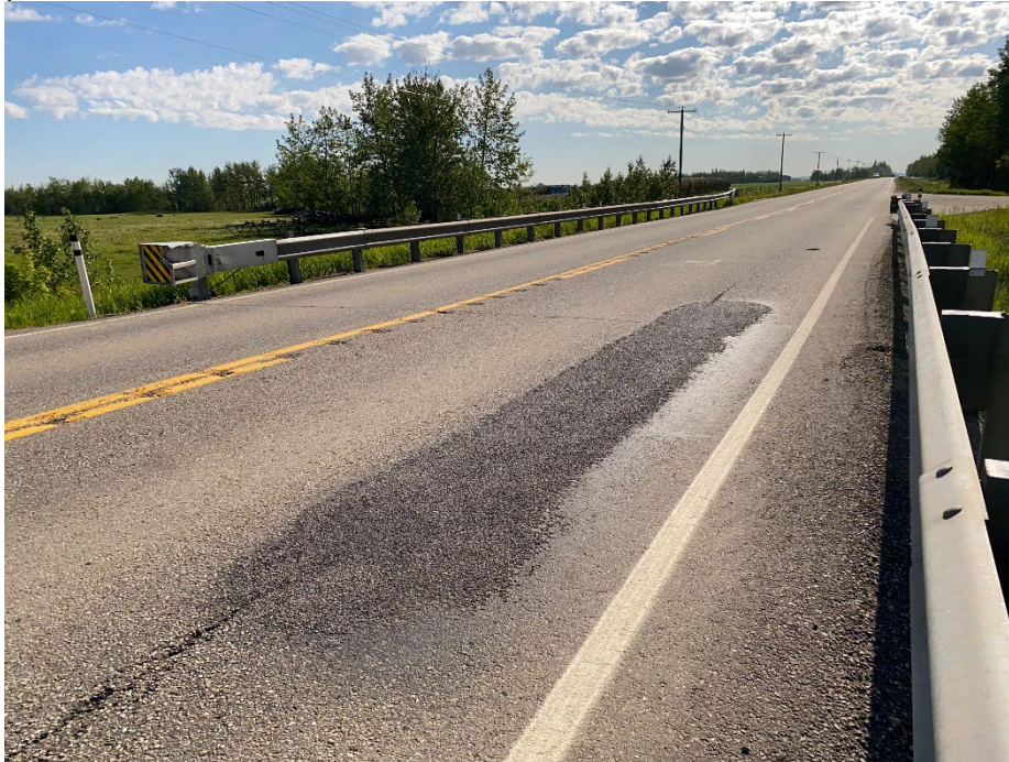
Photo 5: Highway surface above culvert. Looking east.
