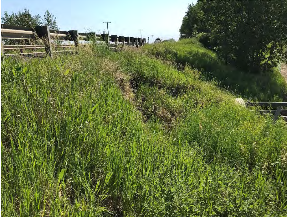
Photo 3: Scarp at west slump. Looking east.
