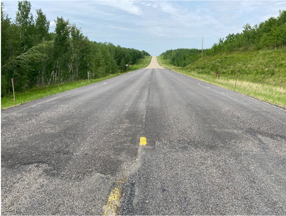
Photo 1: Pavement recently patched in Fall 2022. Looking north.
