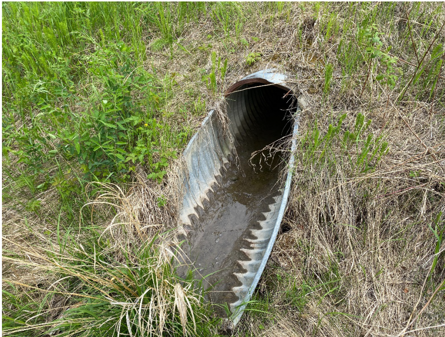
Photo 6: No flow at culvert outlet but wet sediment present. Looking southeast.
