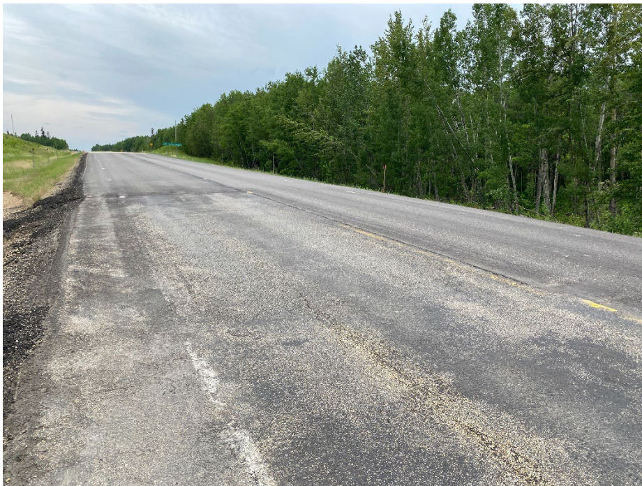
Photo 2: Pavement recently patched in Fall 2022. Looking south.
