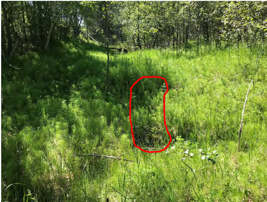
Photo 5: Subsidence along culvert. Looking south.
