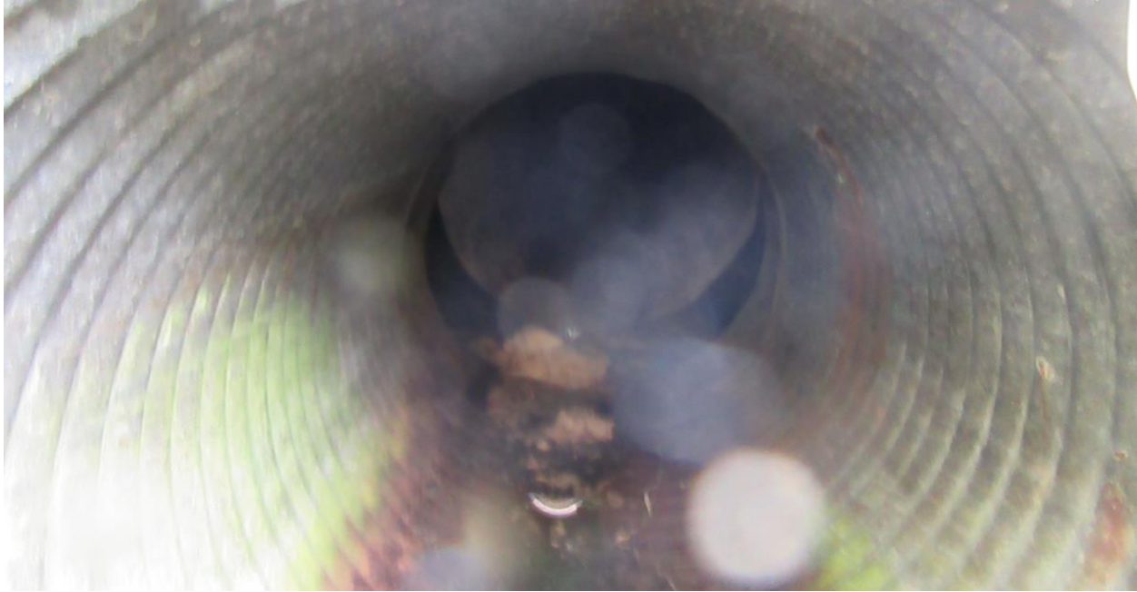
Photo No. 10 – Culvert outlet location: culvert is separated at 4 m from outlet.
