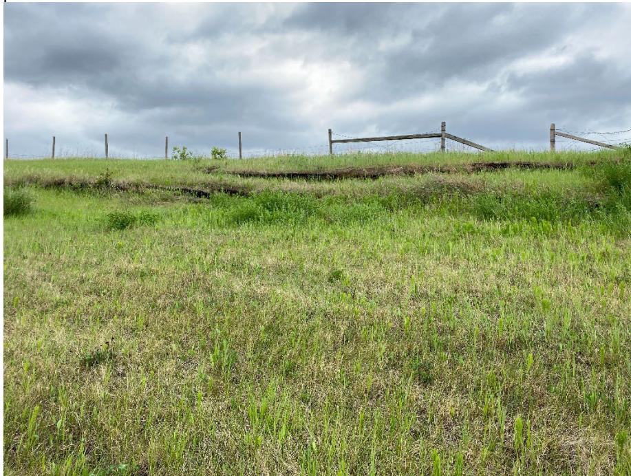
Photo 1: Overall view of scarps on upper slope. Looking south.
