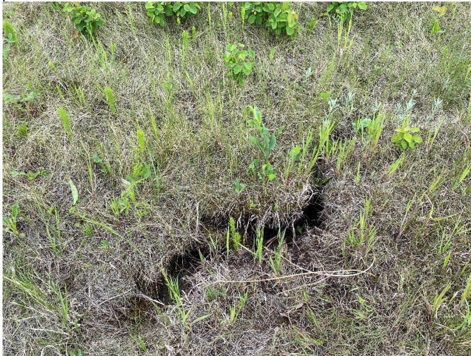
Photo 3: Ground crack downslope from scarps. Looking south.
