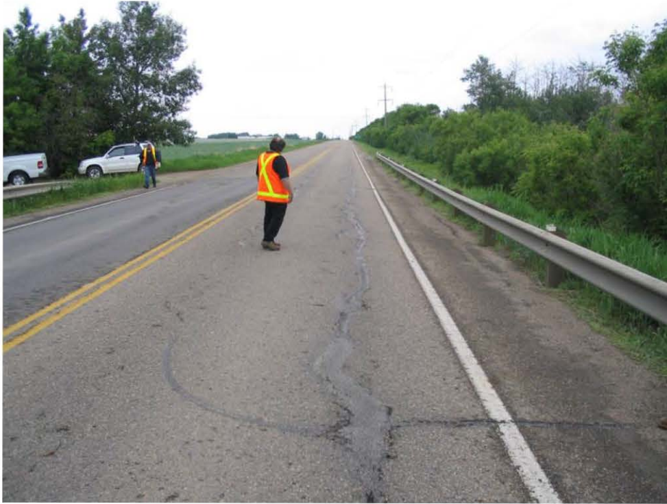
Photo 1 - Looking north at longitudinal crack along pavement, June 7, 2006.
