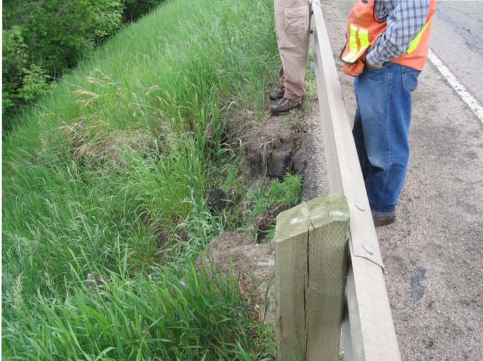
Photo 1 - Looking north at longitudinal crack along pavement, June 7, 2006.
