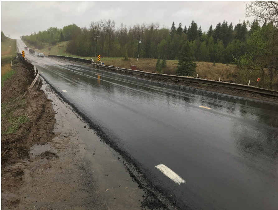
Photo 1: Highway 825. Looking southwest.
