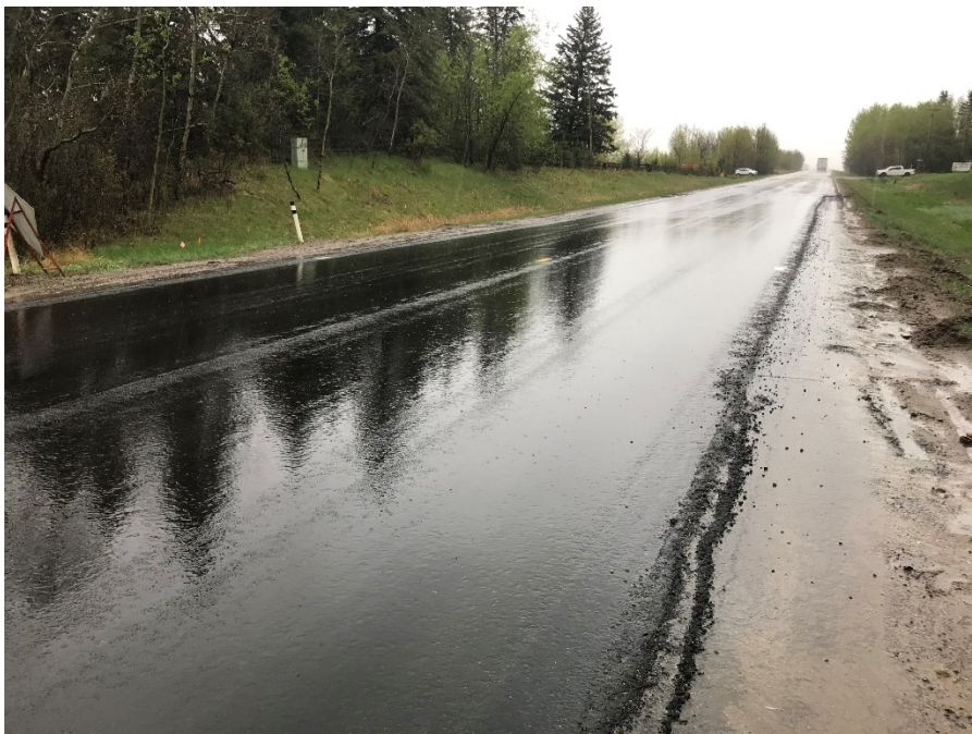
Photo 2: Highway 825. Looking northwest.
