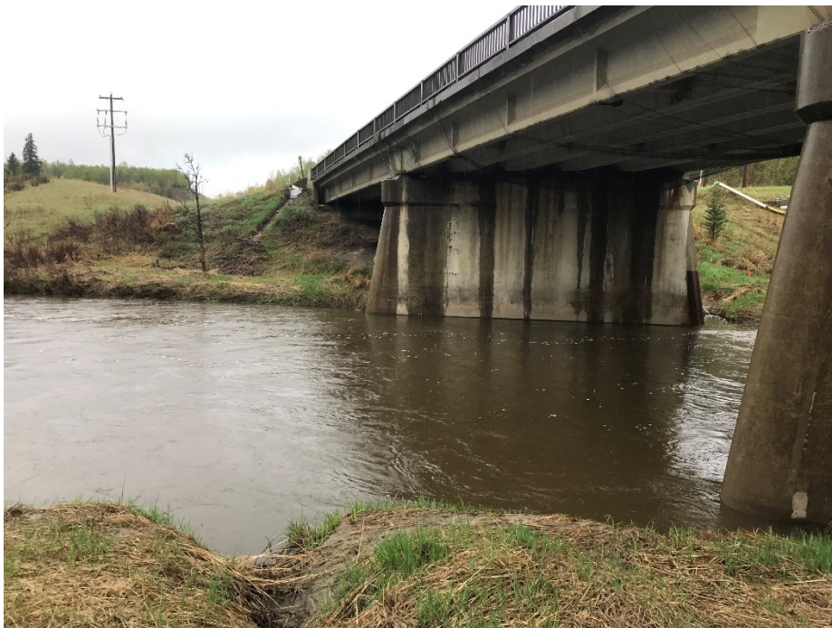
Photo 6: Bridge appeared unaffected. Looking south.
