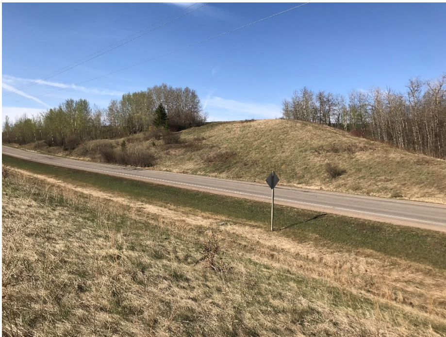
Photo 6: Well vegetated backslope obscuring previously observed exposed bedrock. Looking southwest.
