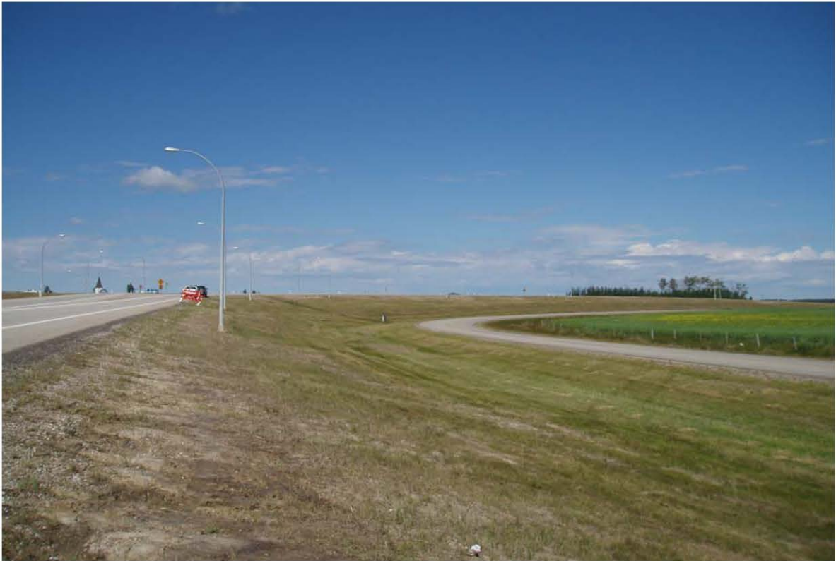
PHOTO 5: West view of the northeast ramp and adjacent service road.
