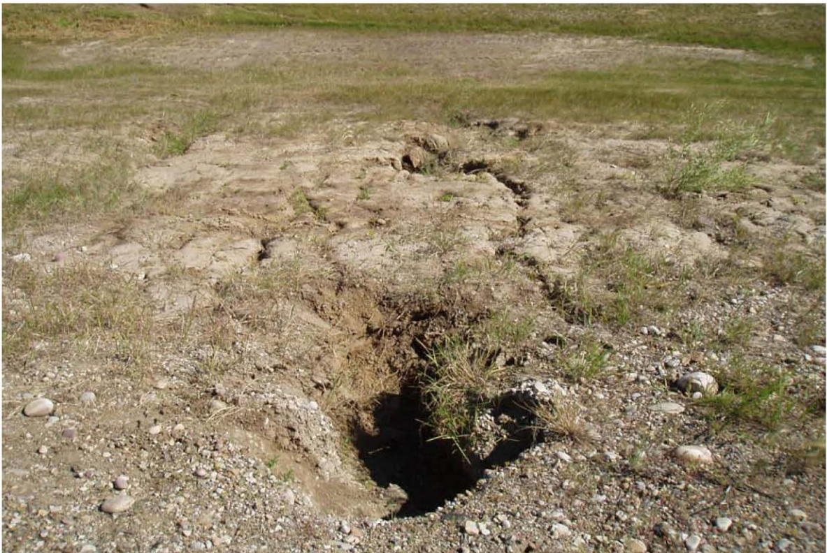
PHOTO 4: View facing downslope of the entrance hole of piping tunnel No. 3, erosion gullies and lack of vegetation.
