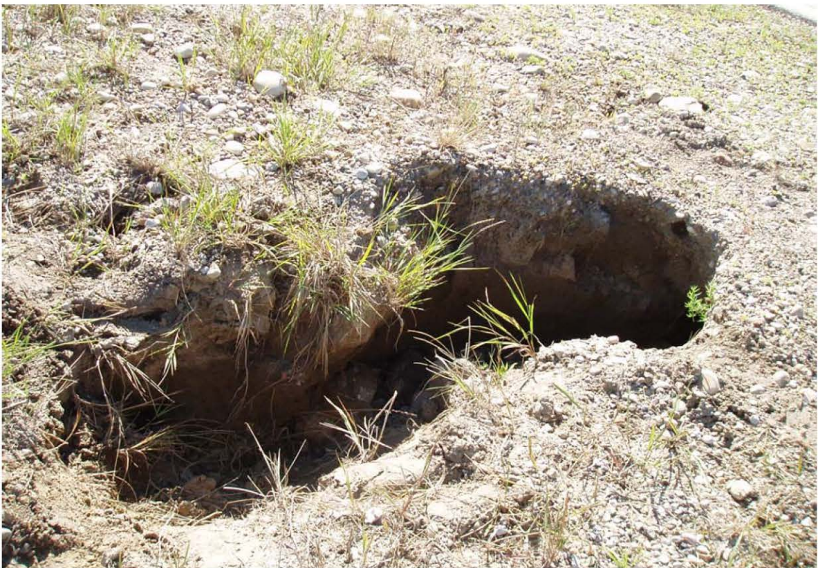
PHOTO 2: Entrance hole of piping tunnel No. 3.
