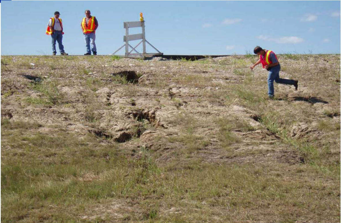
PHOTO 1: View of the north slope of the northeast ramp.
