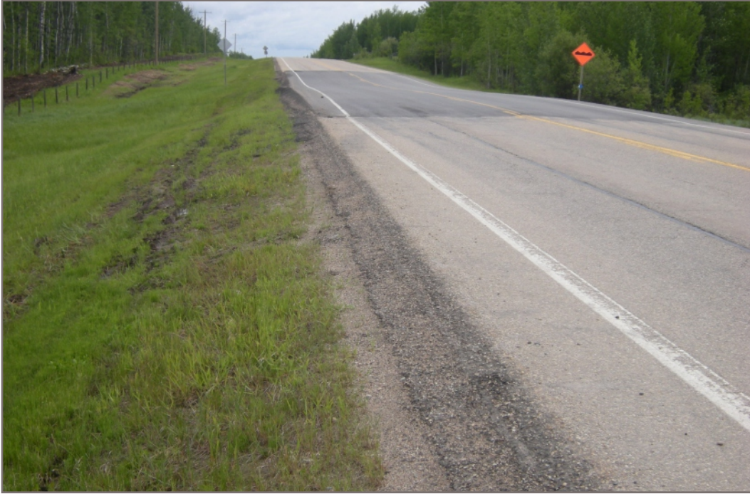
Photo 1: Asphalt overlay placed after foam injection
