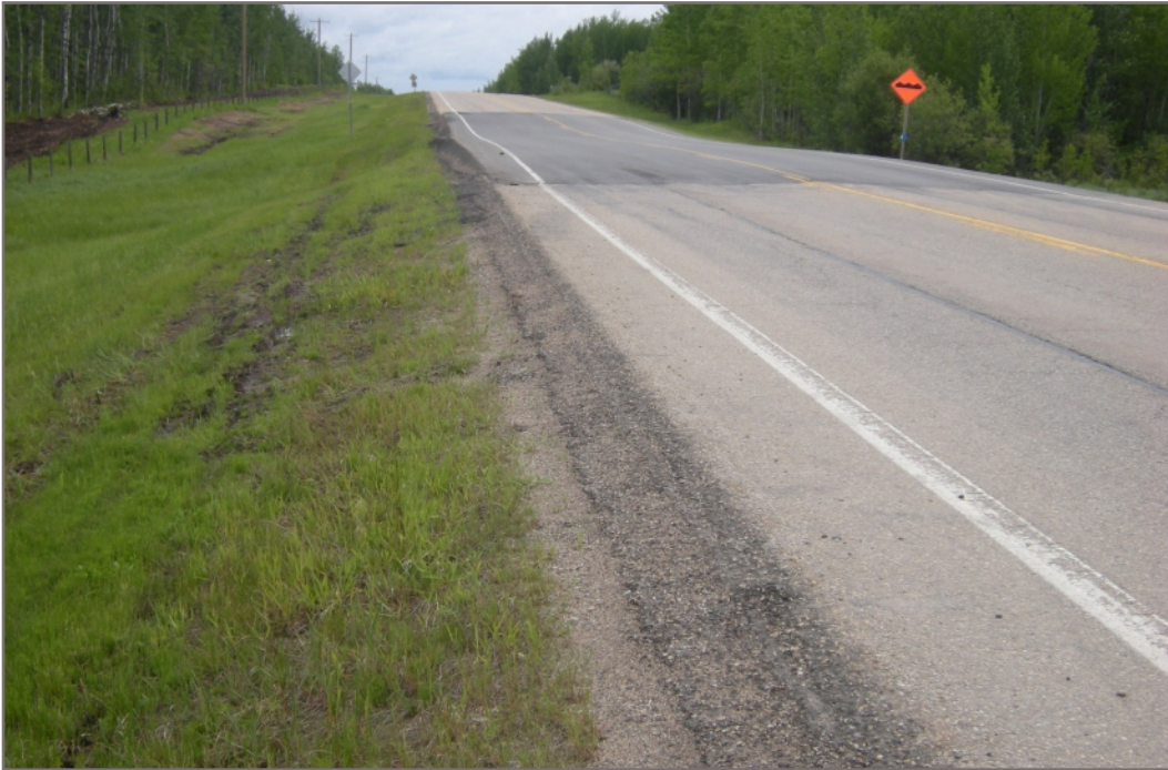
Photo 1: Asphalt overlay placed after foam injection
