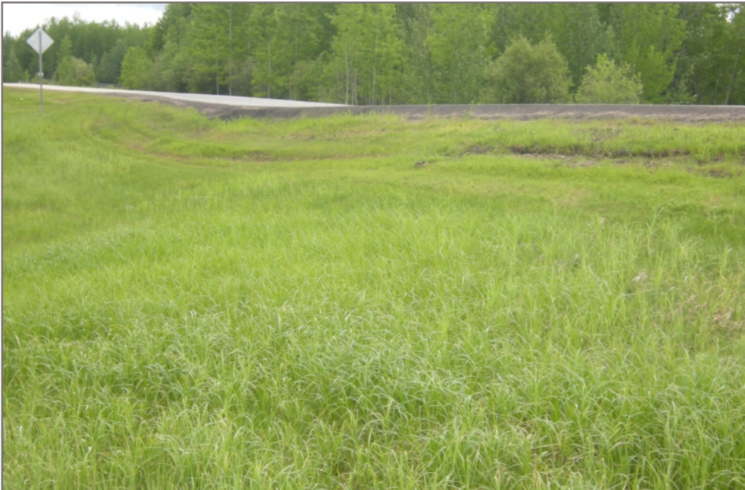
Photo 2: Repaired pavement dip facing northeast
