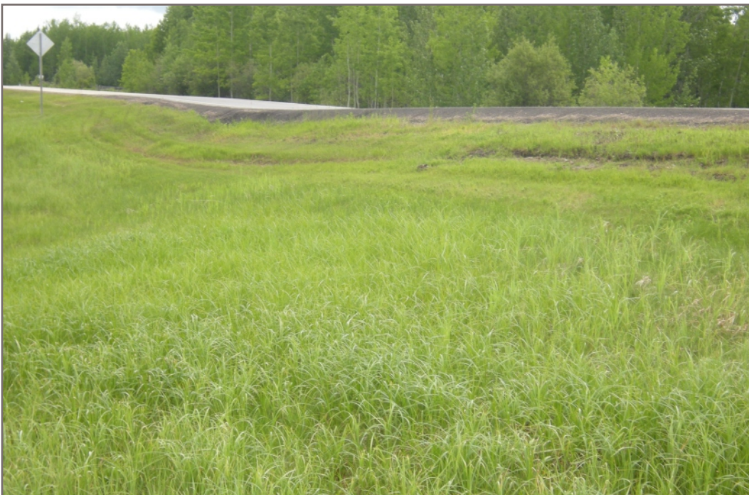
Photo 2: Repaired pavement dip facing northeast
