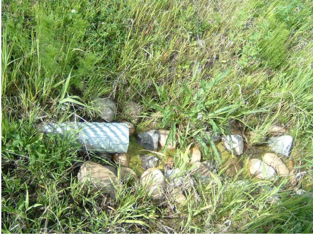
Photo 5 – South end drain outlet (2005).
