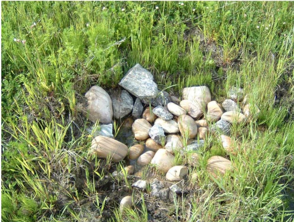
Photo 4 – North end drain outlet (2005).
