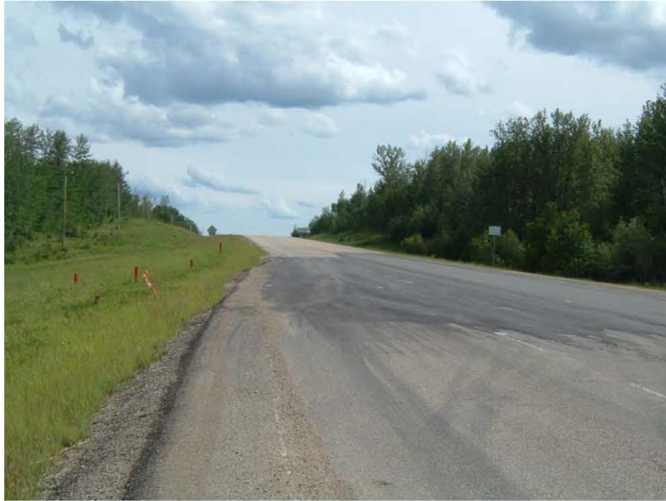
Photo 1 – New overlaid area, looking south (2005).
