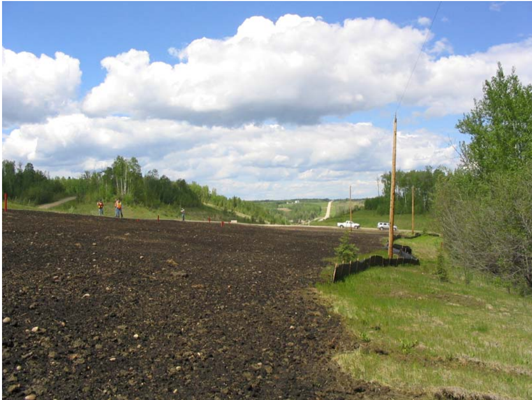
Photo 1. Side slope after pile wall construction.
