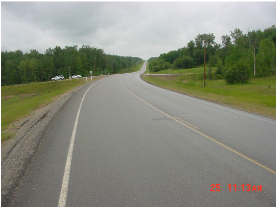
PHOTO NC16-2 LOOKING NORTH FROM SOUTH END OF REPAIR AREA
