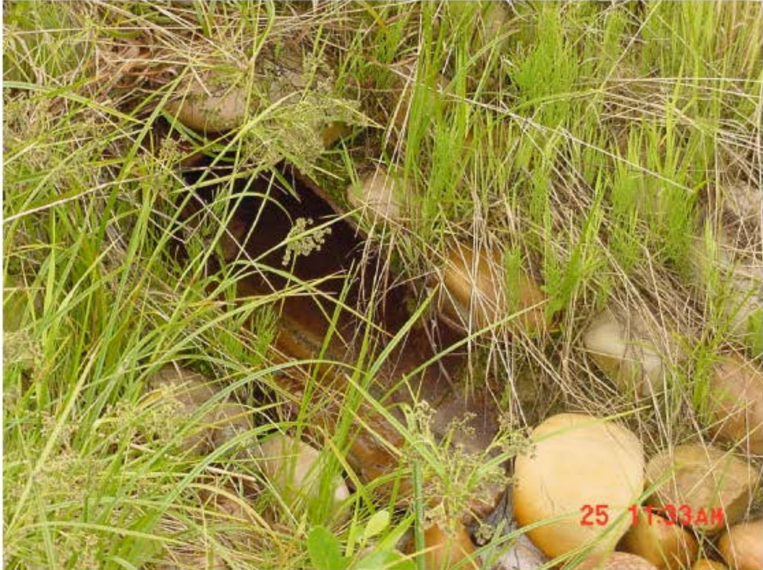
PHOTO NC16-3 CULVERT OUTLET ON WEST SIDE OF EMBANKMENT
