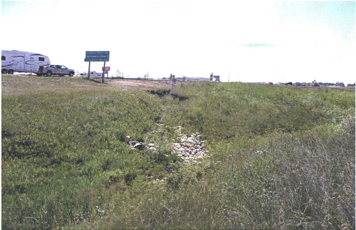
PHOTO 3: Looking southeast at the erosion gully and the transition turn of the ditch. The 900 mm diameter CSP outlet is also visible.
