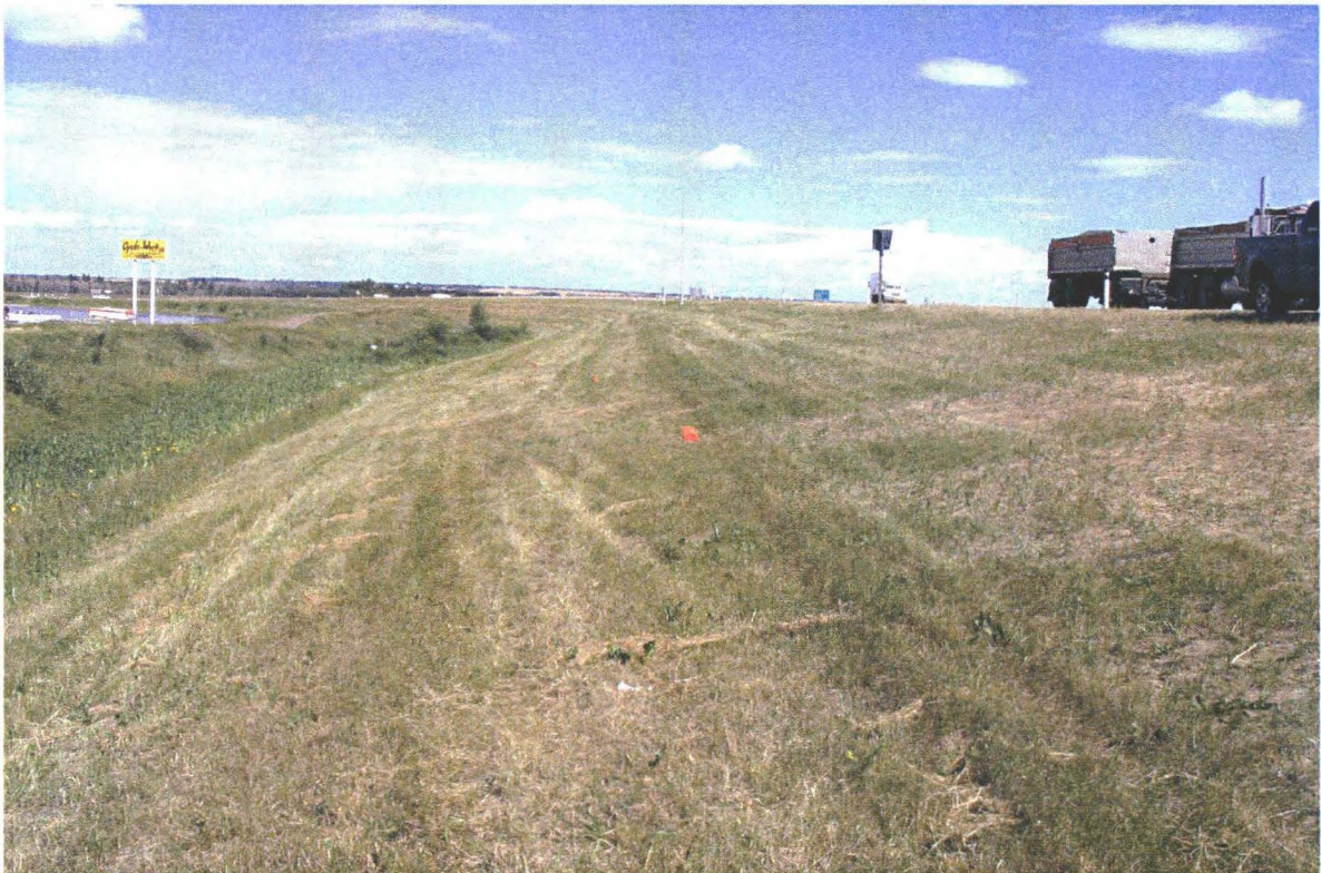
PHOTO 2: View of the lower level highway ditch, looking north.
