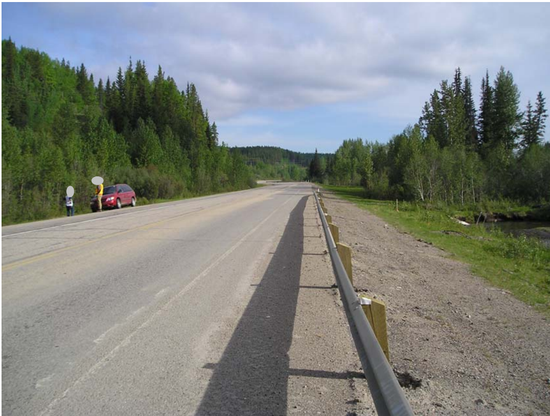
Photo 3 – Looking north along edge of pavement.
