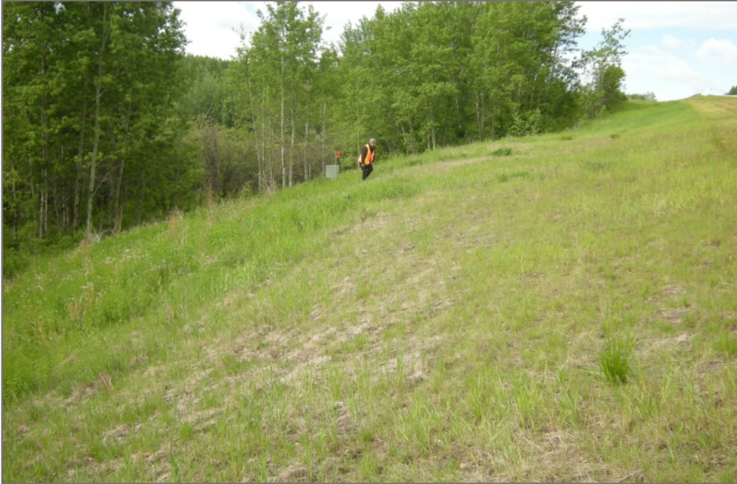
Photo 1: Toe berm (Site B)
