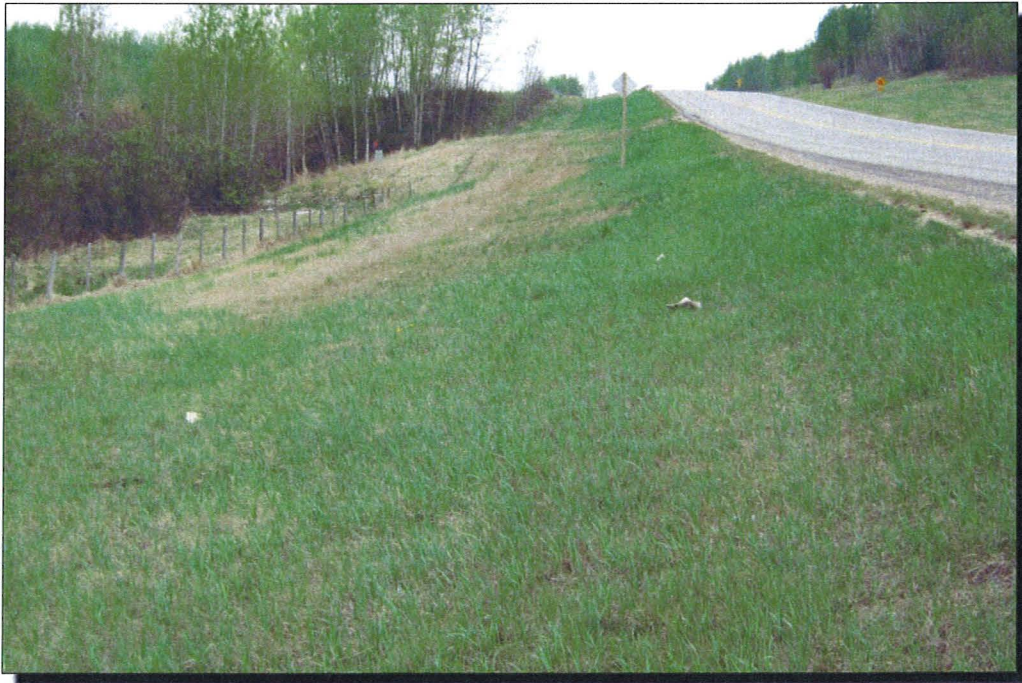
Photo 1 Toe berm site (Site B) located upslope just behind road sign
