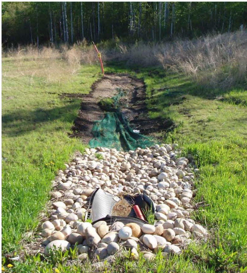
Photo 2. New swale realignment
