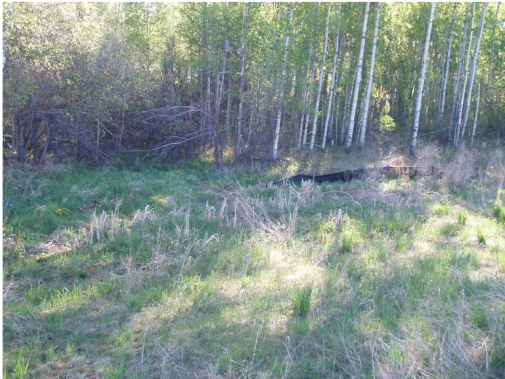
Photo 4 – View of the berm's toe area
