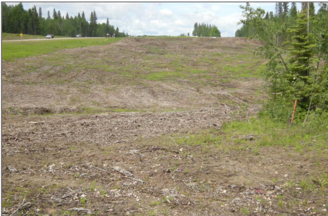
Photo 2: Site clearing in preparation of highway twinning
