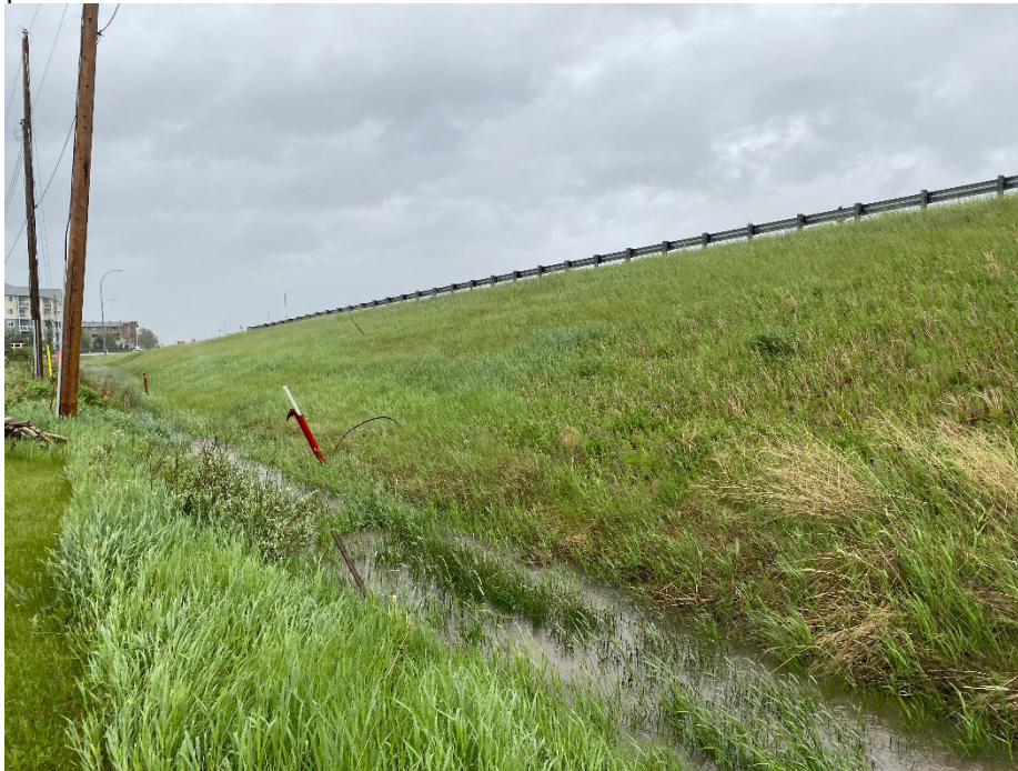
Photo 1: Repaired south slide, looking southwest.
