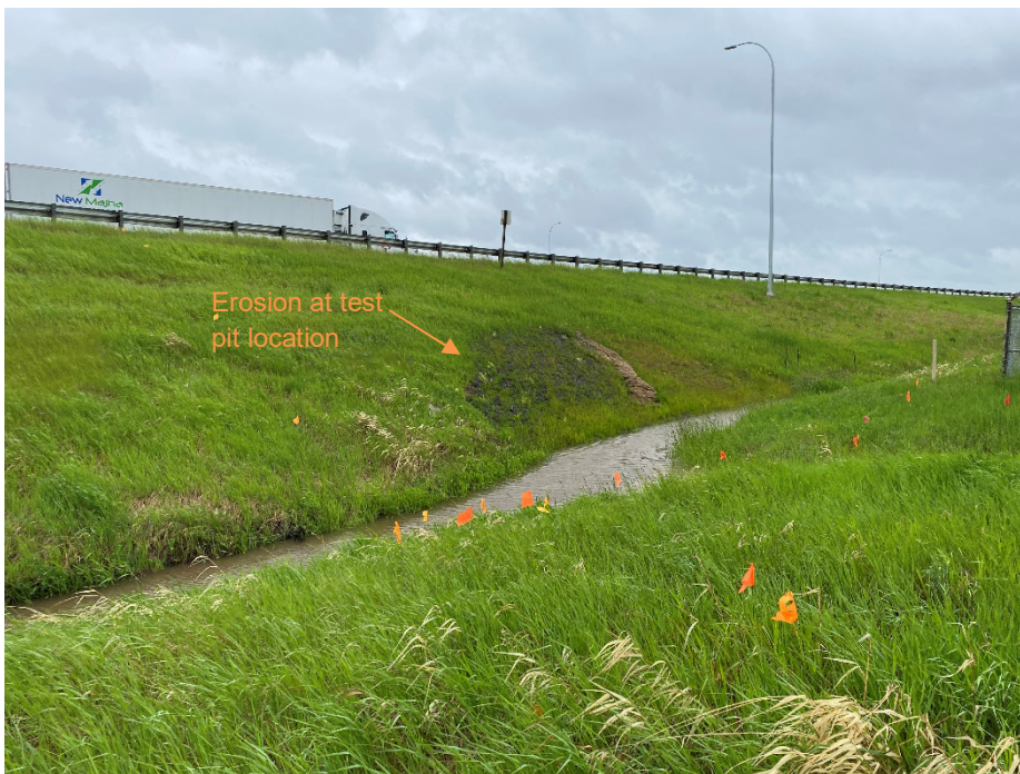
Photo 2: Repaired test pit area, looking northwest.
