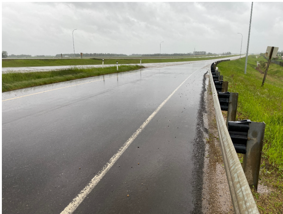
Photo 6: On-ramp to Highway 2 north bound. Looking northwest.
