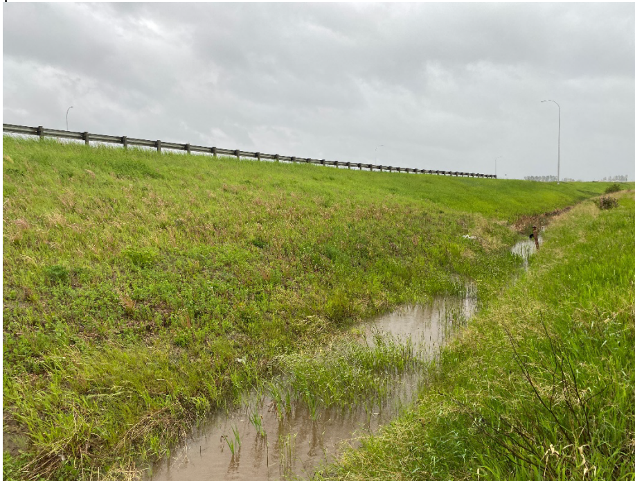
Photo 2: Repaired north slide, looking northwest.
