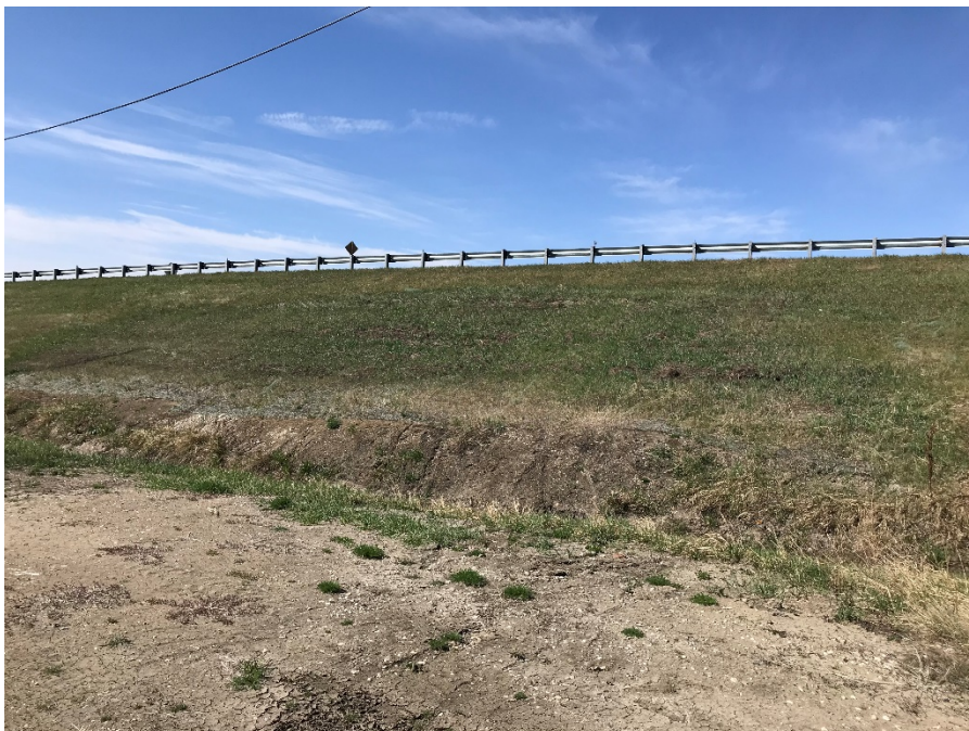
Photo 2: Repaired south slump. Looking west.
