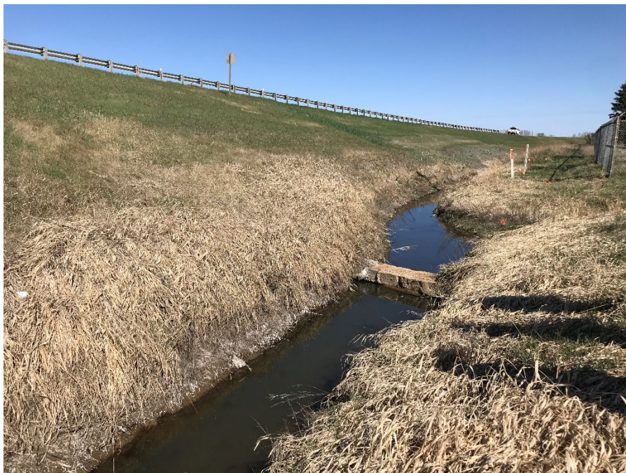
Photo 6: Cleaned and de-vegetated ditch. Looking north.
