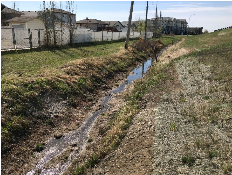
Photo 5: Cleaned and de-vegetated ditch. Looking south.
