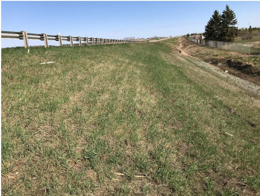
Photo 1: Repaired north slide. Looking north.
