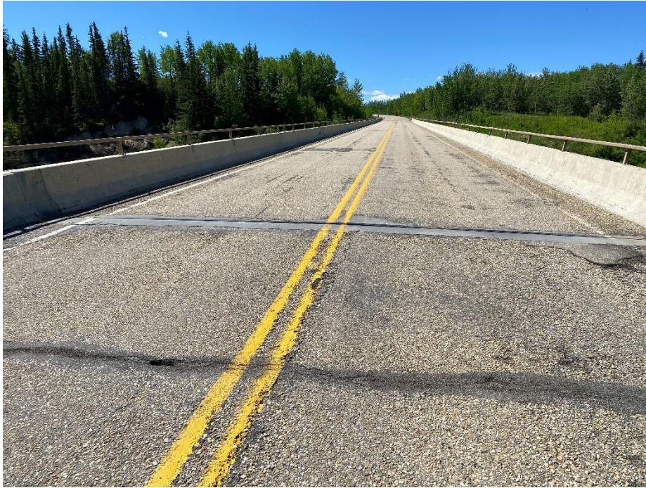
Photo 1: Highway surface at north abutment. Looking southwest.
