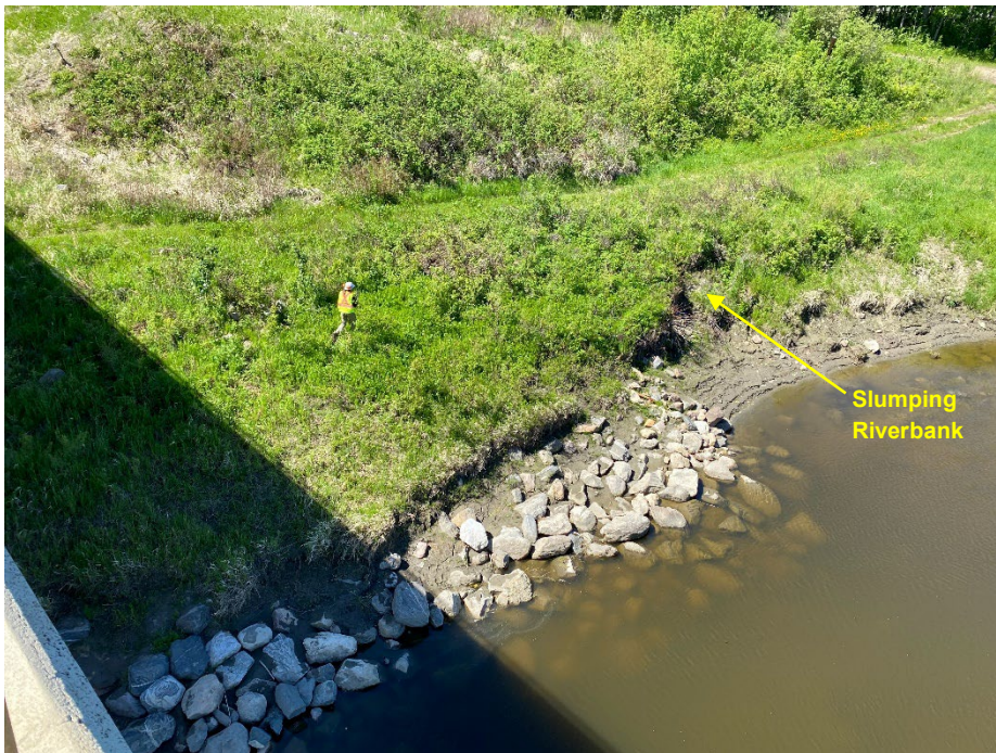
Photo 10: Upstream side of south abutment. Looking southwest.
