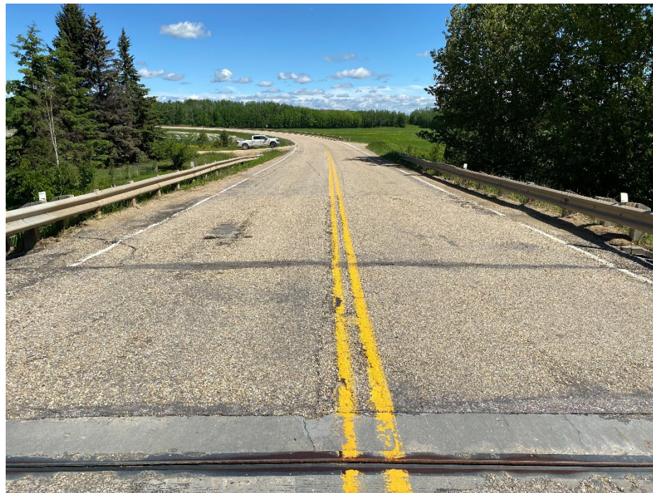
Photo 2: Highway surface at north abutment. Looking northeast.
