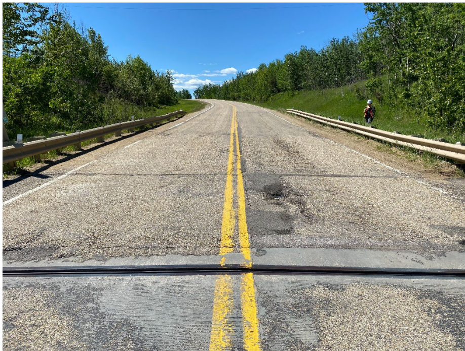
Photo 4: Highway surface at south abutment. Looking southwest.
