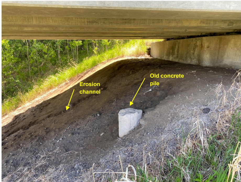
Photo 11: South abutment head slope. Looking east.
