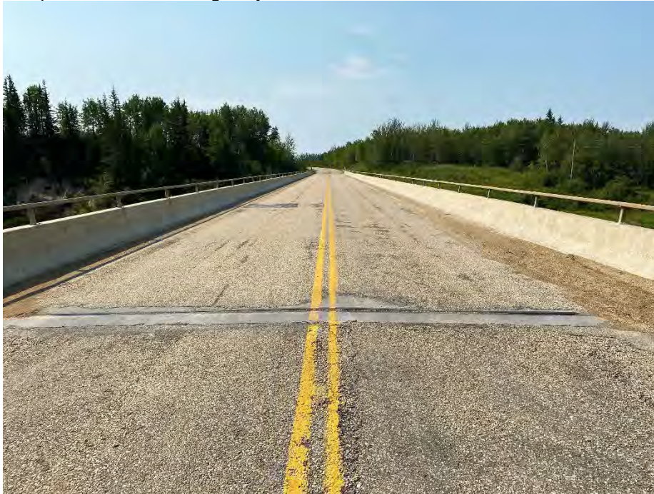
Photo 1: Highway surface at north abutment. Looking southwest.
