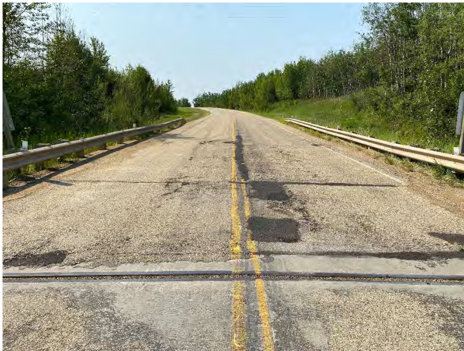
Photo 4: Highway surface at south abutment. Looking southwest.
