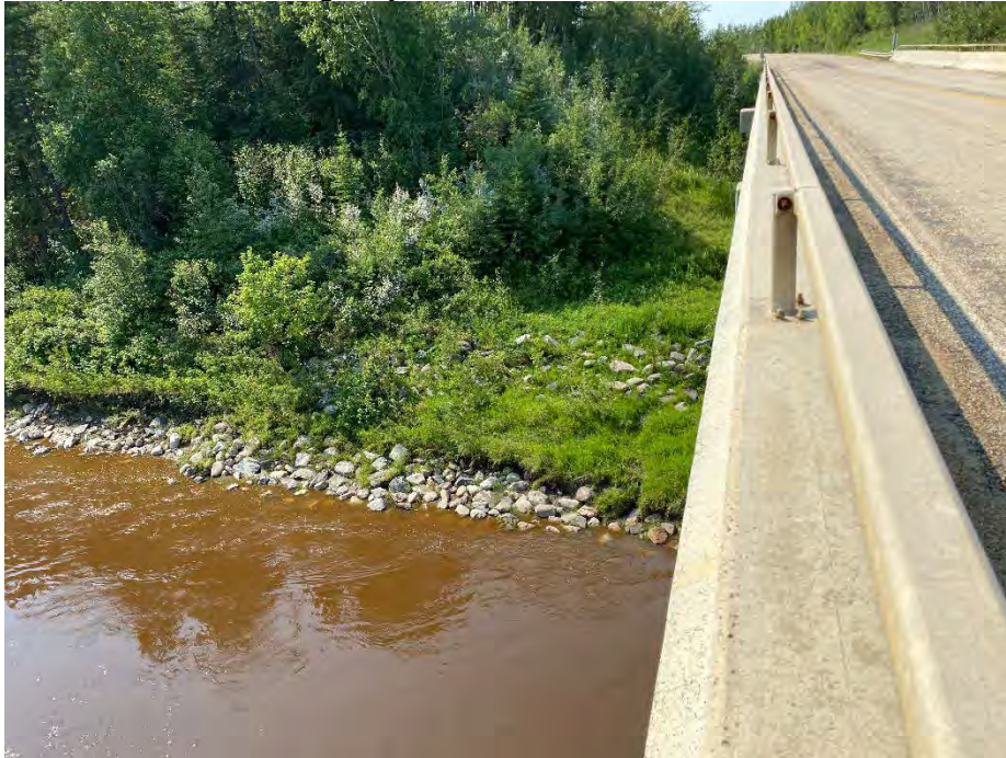
Photo 9: Downstream side of south abutment. Looking southeast.
