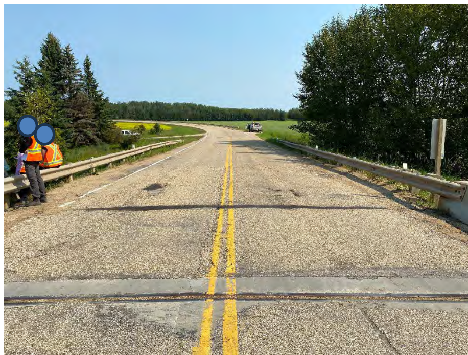
Photo 2: Highway surface at north abutment. Looking northeast.
