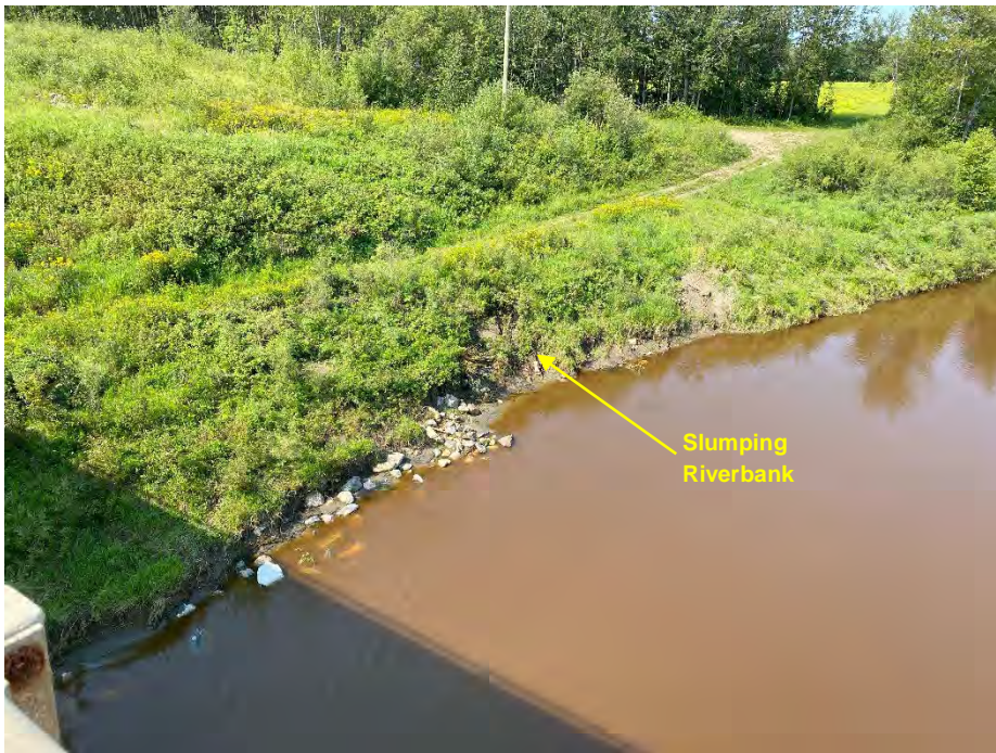
Photo 10: Upstream side of south abutment. Looking southwest.
