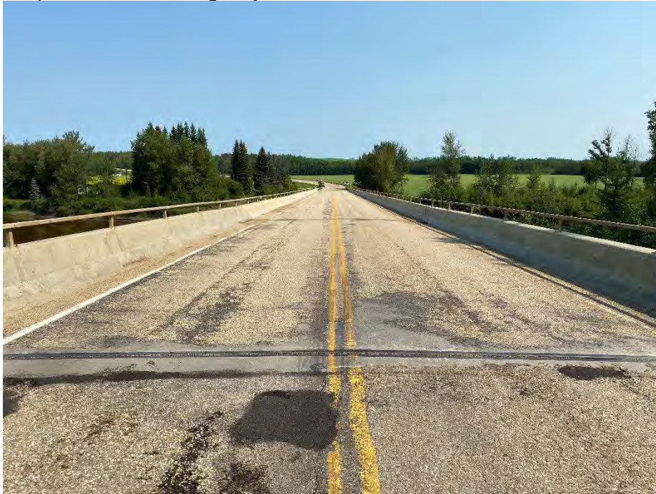
Photo 3: Highway surface at south abutment. Looking northeast.
