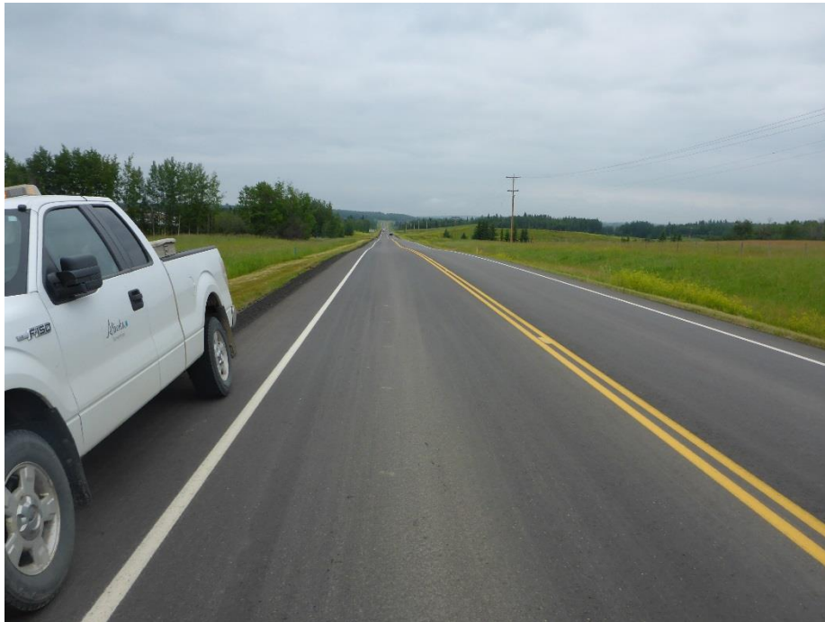
Photo 1: Pavement recently overlayed. Looking north.
