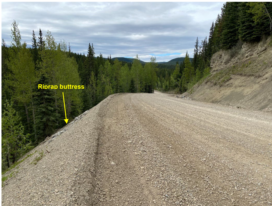
Photo 6: North end of washed-out NBL. Looking south.
