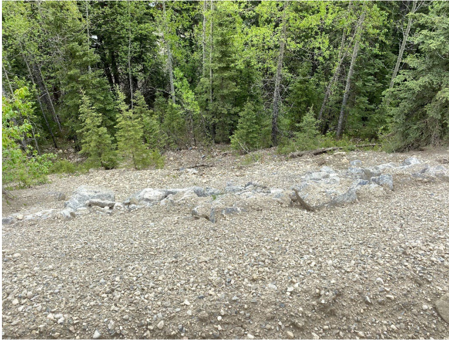
Photo 7: Riprap buttress constructed at location of NBL wash-out repair. Looking southeast.
