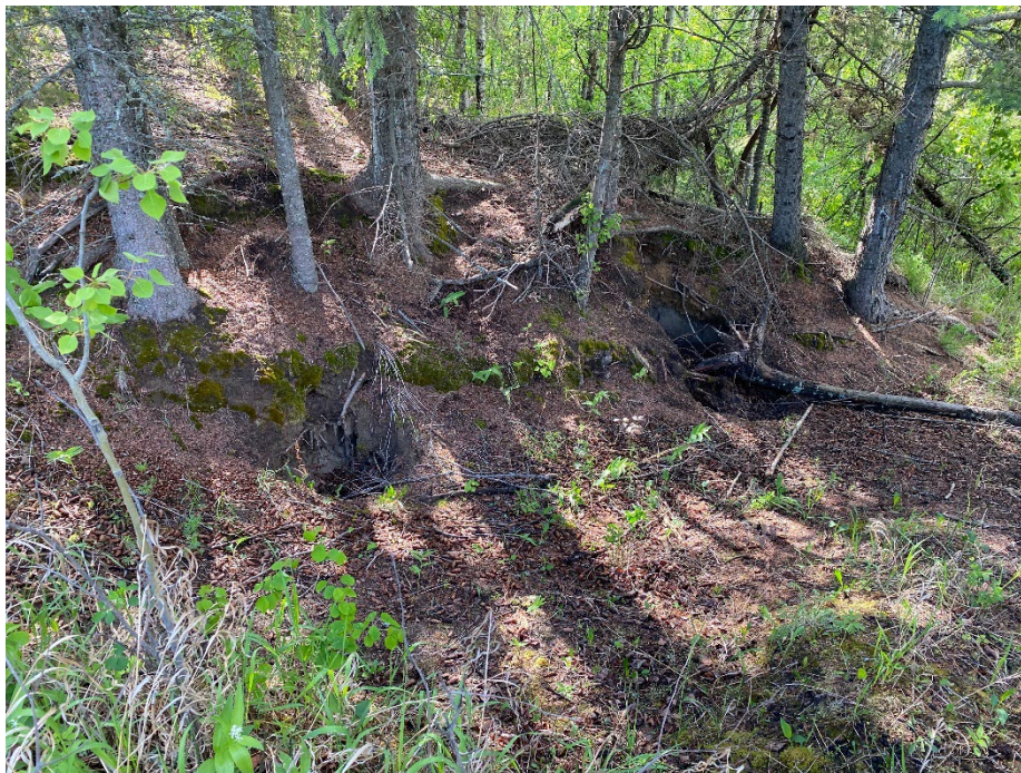
Photo 6: Two sinkholes in ravine. Looking southeast.
