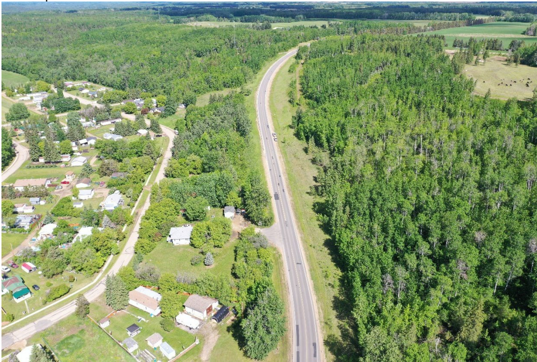
Photo 9: Site overview, taken by drone. Darker pavement patches are deficiency repairs, approx. 2 weeks old at time of photo. Looking northwest.
