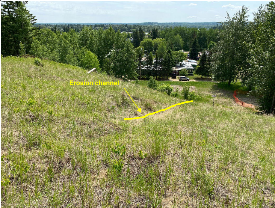
Photo 7: Sand exposed in erosion channel heading downslope to the bench. Looking southwest.
