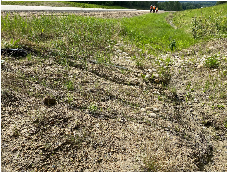
Photo 1: Erosion gully through the old ditch block with erosion rills into the ditch. Looking south.
