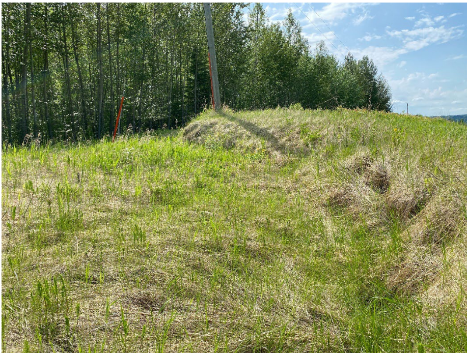
Photo 6: Old scarp and leaning power pole. Looking southeast.
