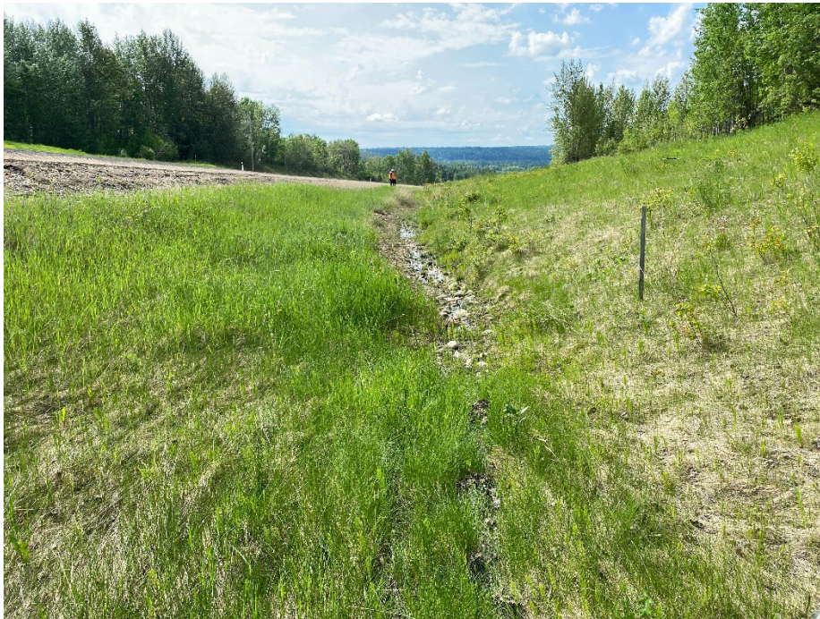
Photo 4: West ditch south from the old ditch block with gulying and exposed cobbles. Looking south.
