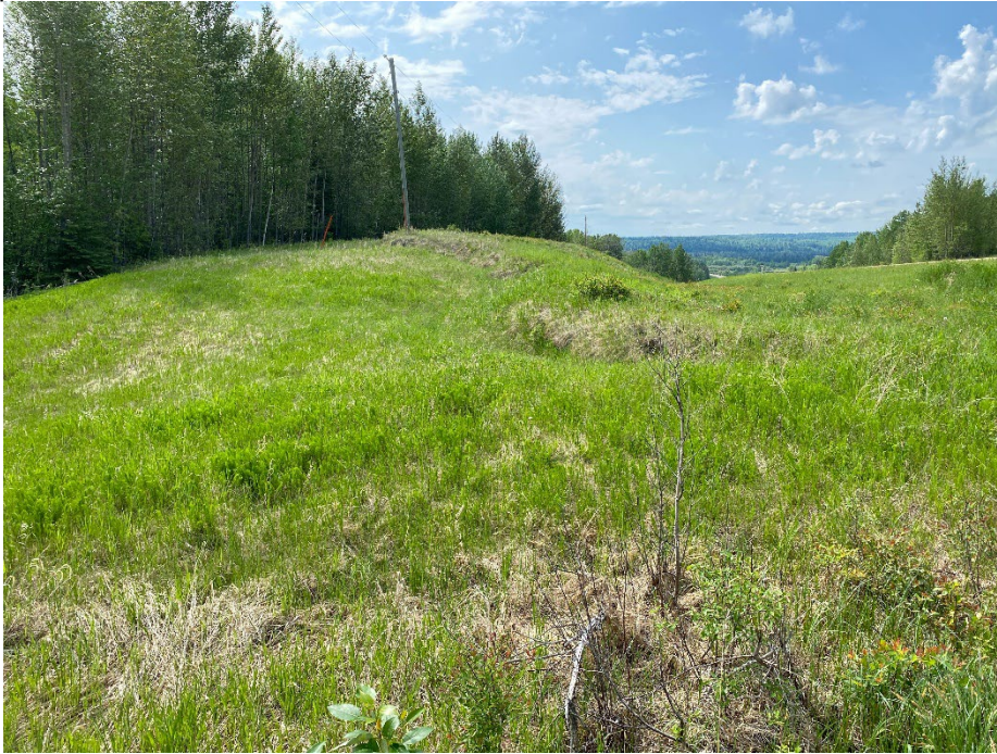
Photo 5: Old landslide east of Highway 658, looking south.
