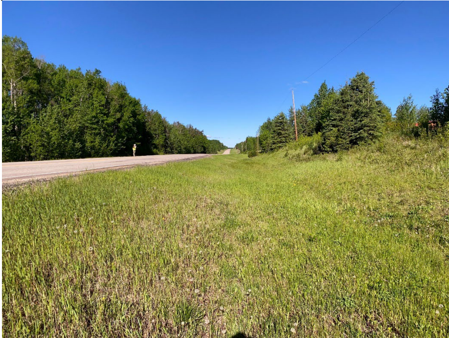
Photo 5: Ditch and embankment on north side of highway. Facing west.
