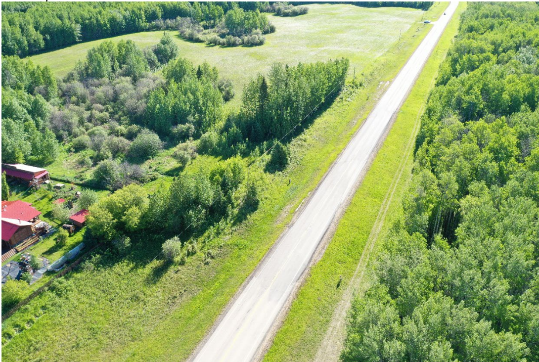
Photo 7: Site overview, taken by drone. Looking northeast.
