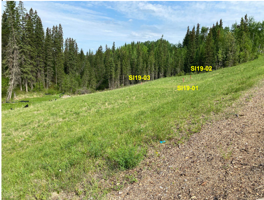
Photo 5: Repaired slope and berm location. Looking northwest.
