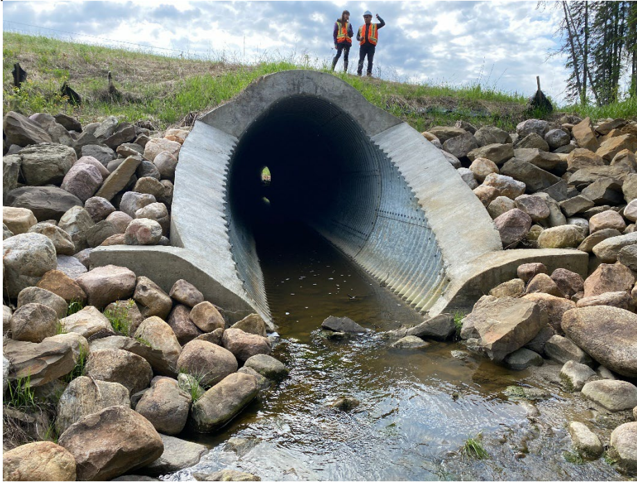
Photo 3: Culvert outlet, looking southeast.
