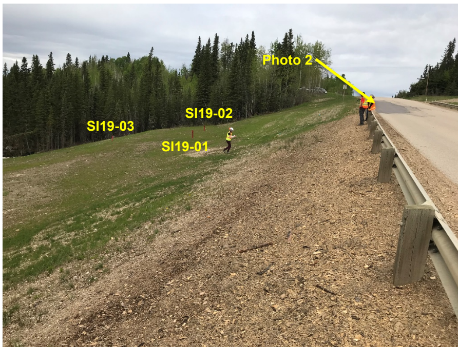
Photo 6: Repaired slope and berm location. Looking north.
