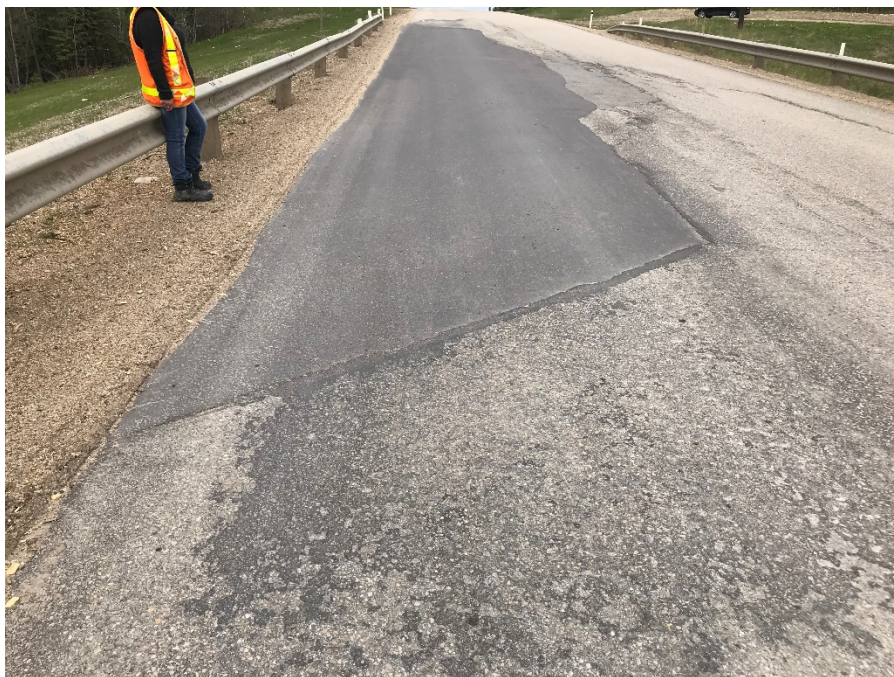
Photo 2: Repaired portion of Highway 658. Looking north.
