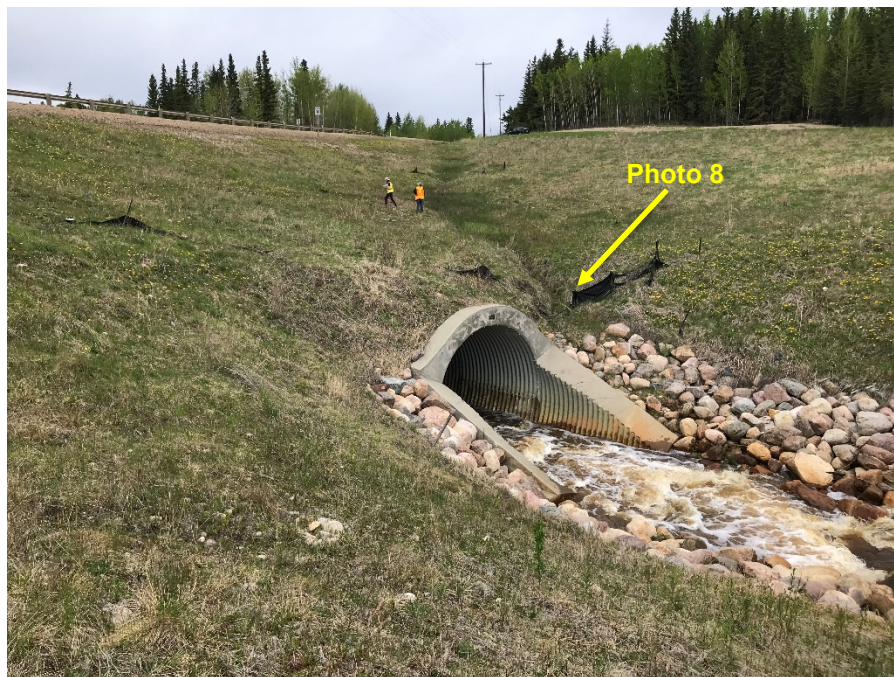
Photo 7: Erosion along drainage ditch to culvert inlet. Looking north.
