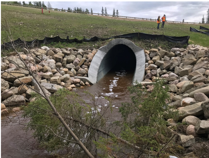
Photo 4: Repaired culvert. Looking southeast.
