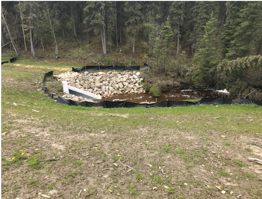
Photo 3: Culvert extended downstream. Looking southwest.
