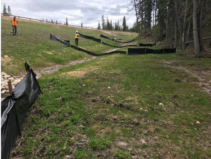
Photo 5: Regraded swale leading to culvert outlet. Looking southeast.
