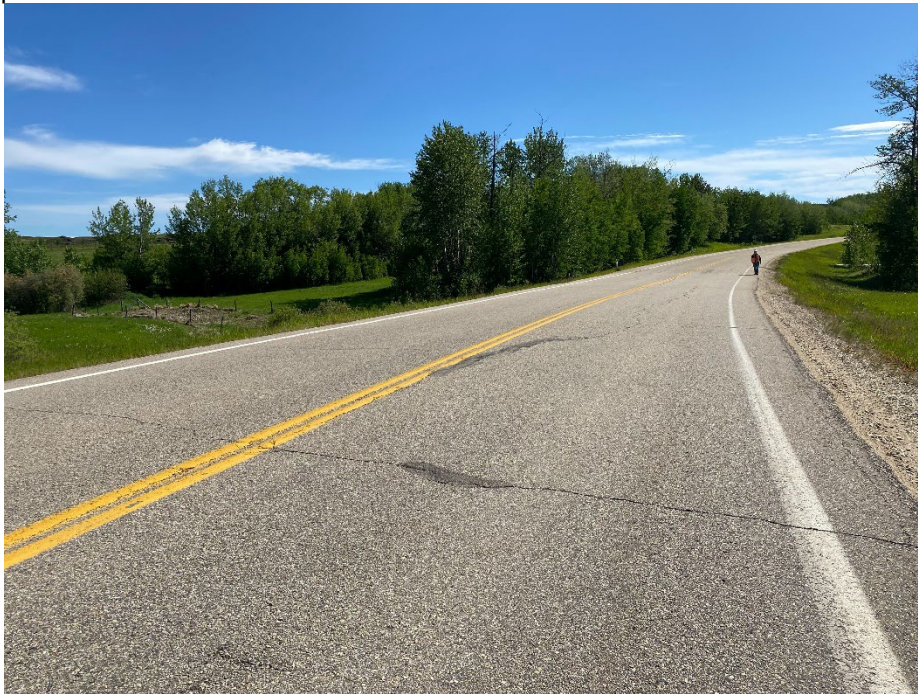
Photo 5: Semi-circular crack along C/L and EBL lane north of BH17-01. Transverse cracking. Looking east.
