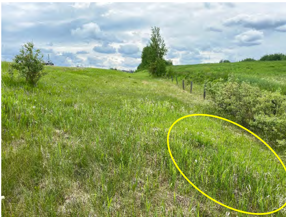
Photo 8: Slumping in north ditch, north from BH17-01. Looking southwest.
