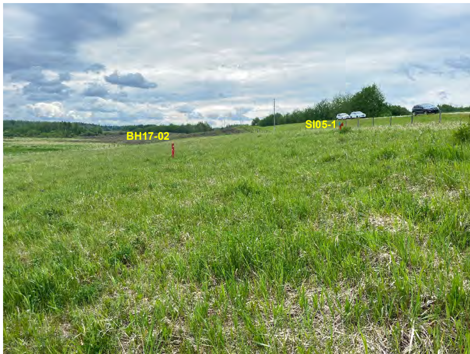
Photo 6: South toe berm. Looking west.
