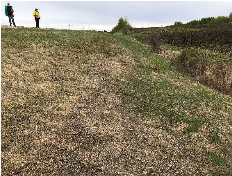
Photo 6: Overall view of north side of highway embankment. Looking west.
