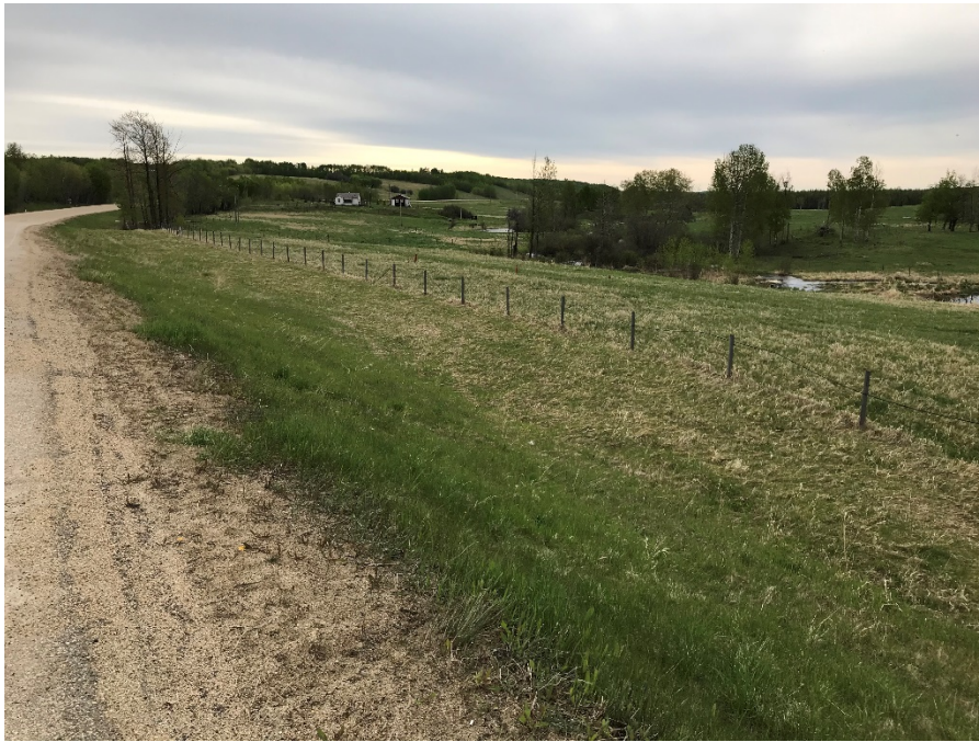
Photo 7: Overall view of south side of highway embankment. Looking east.
