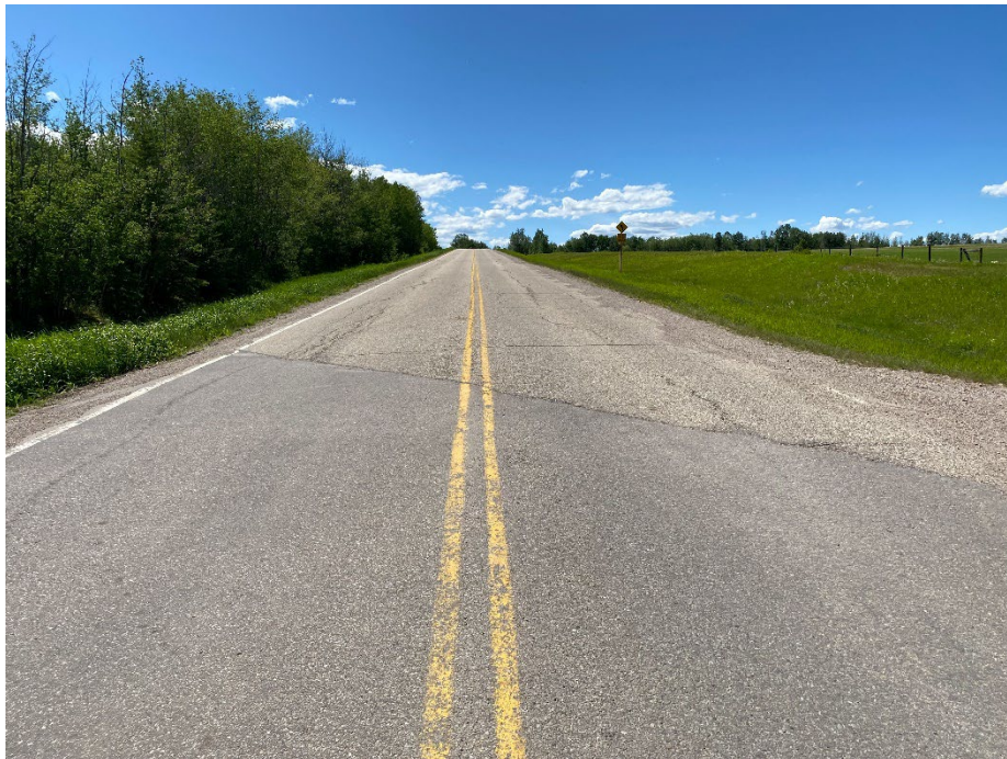
Photo 2: Pavement repair along Highway 16A. Looking west.
