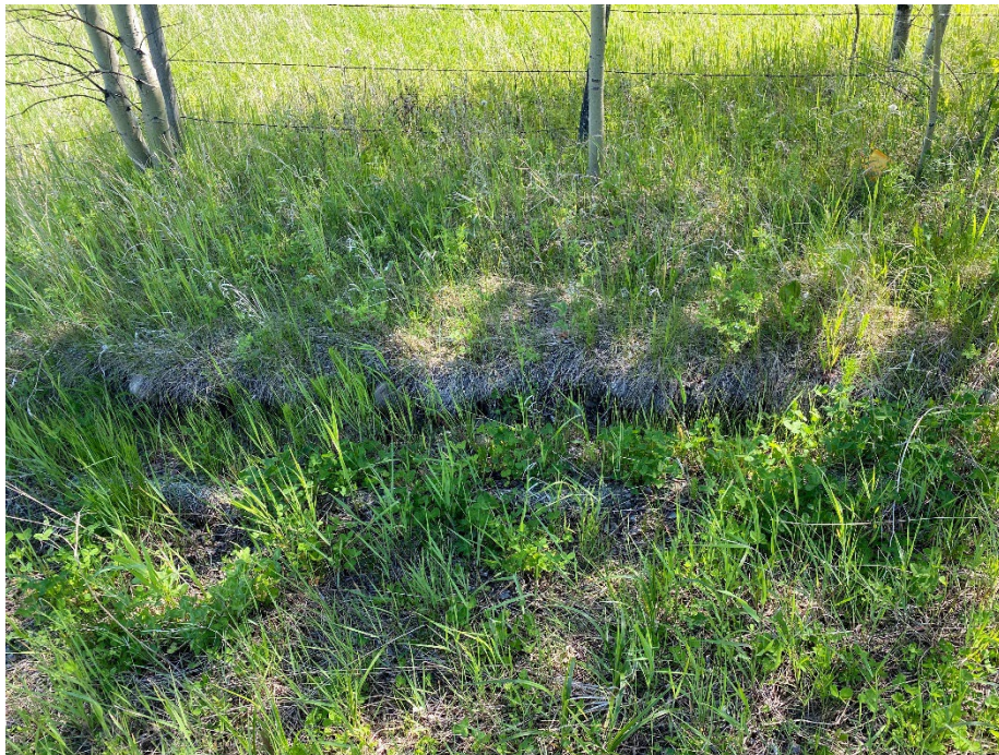
Photo 6: Possible ground crack in south ditch near fence line. Looking south.
