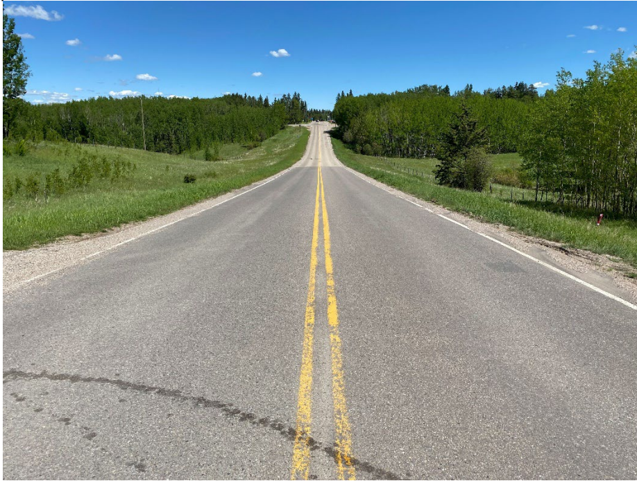
Photo 1: Pavement and embankment repair along Highway 16A. Looking east.
