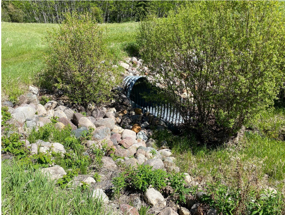
Photo 7: Culvert on south side of highway. Looking southeast.
