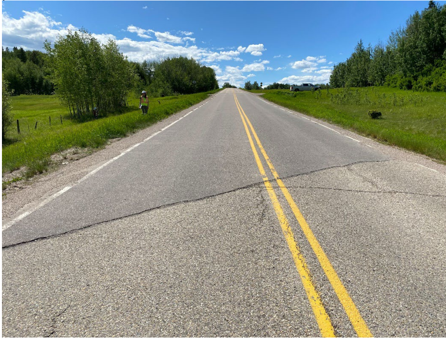
Photo 3: East end of repair zone. Looking west.
