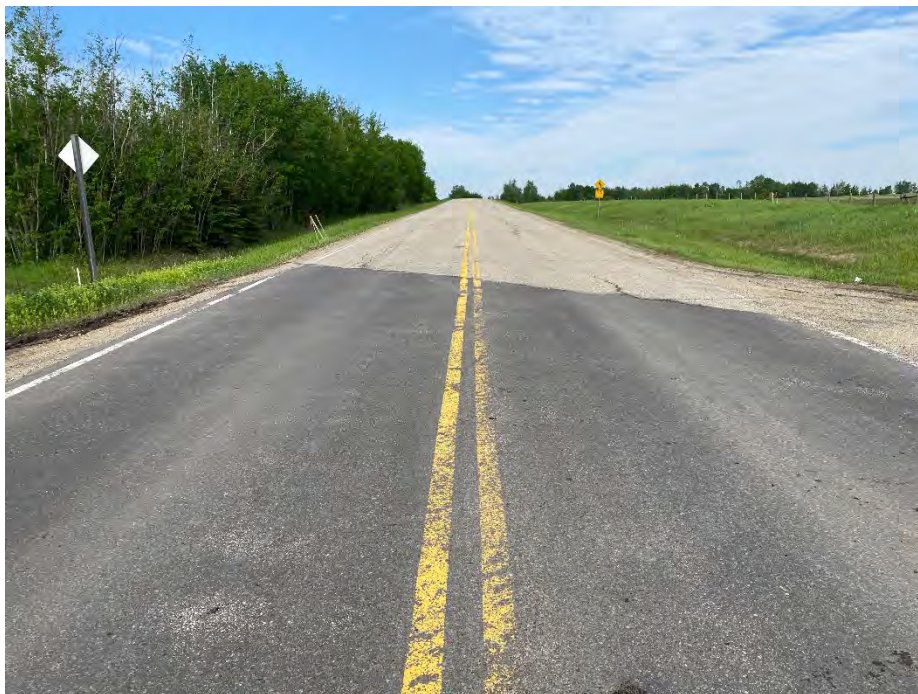
Photo 2: Pavement repair along Highway 16A. Looking west.
