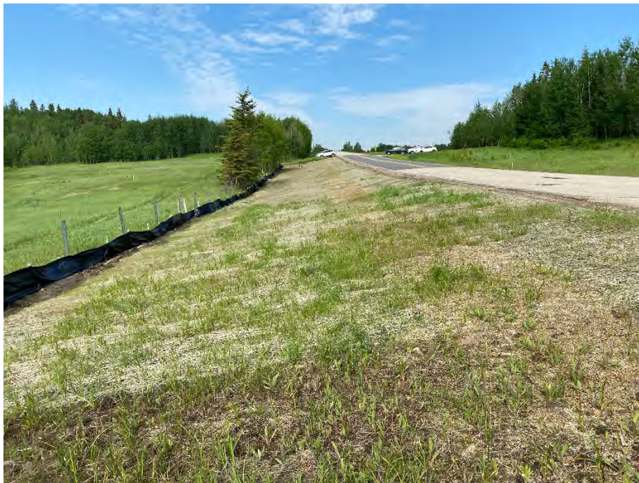
Photo 4: South embankment. Looking west.
