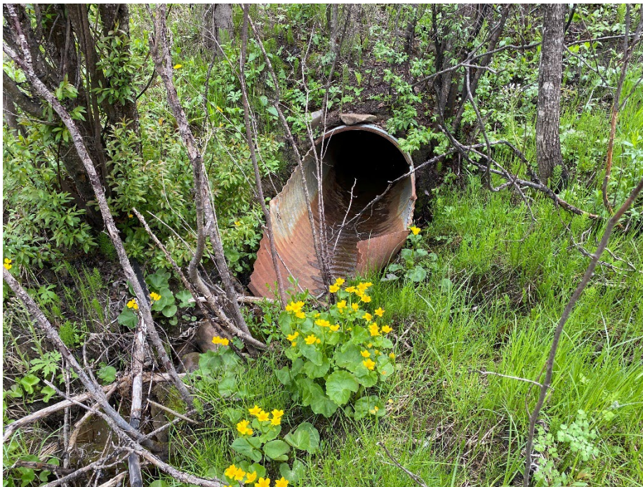
Photo 8: Outlet of 760 mm culvert. Looking southeast.
