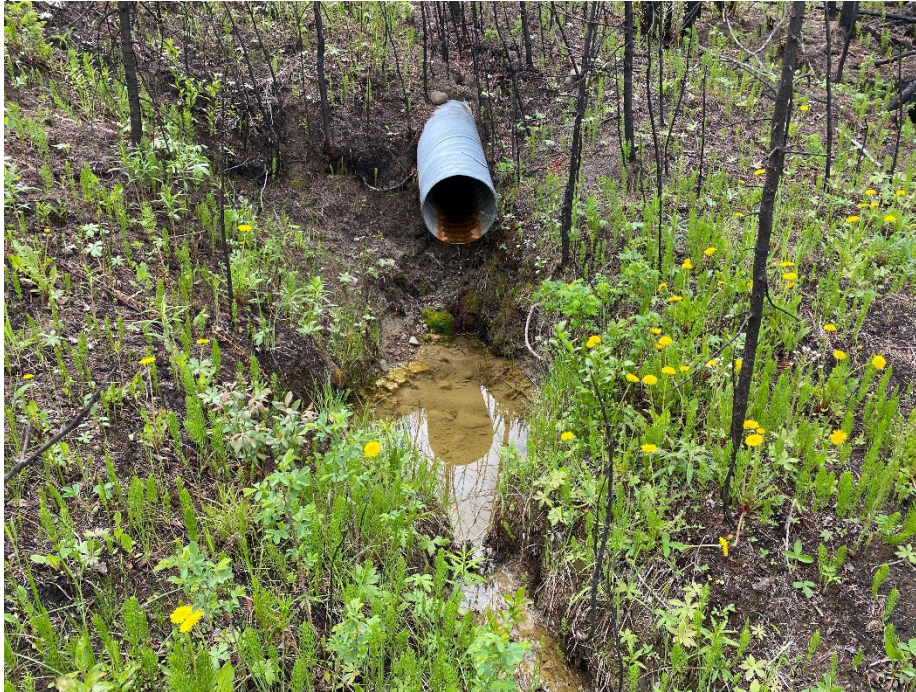
Photo 7: Outlet of 400 mm down drain. Looking south
